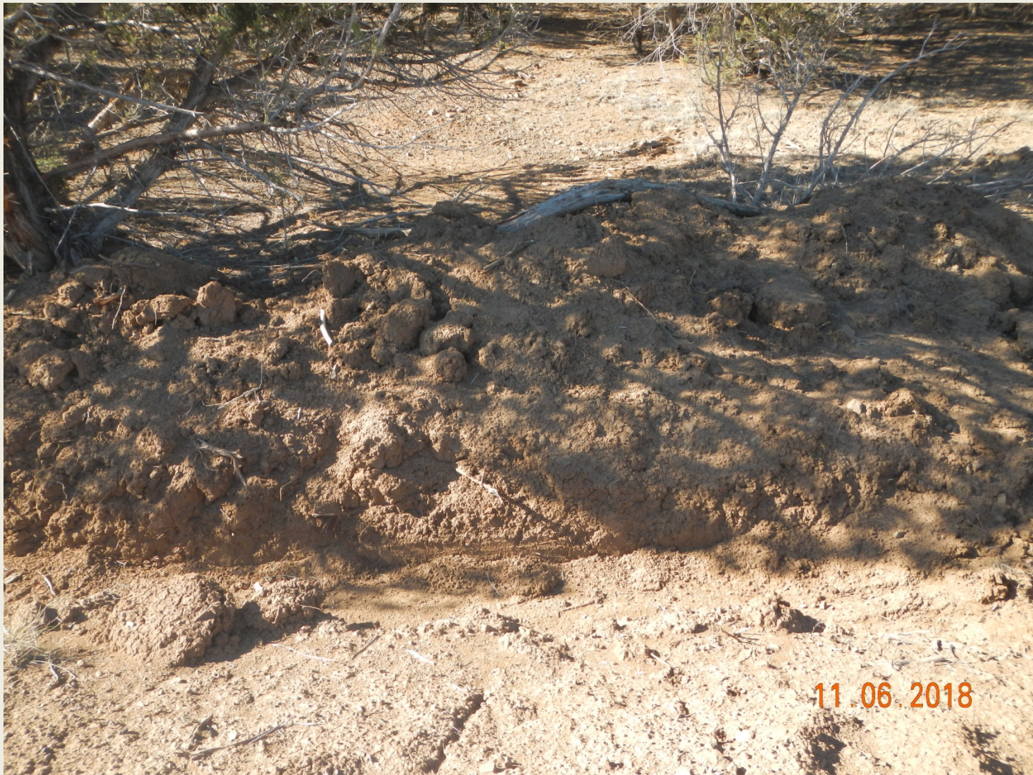
Photo 6. View of unstabilized soils in the northern project area diversion that appear to be discharged from ditch excavation. Erosion control measures such as revegetation need to applied to loose, disturbed soils.
