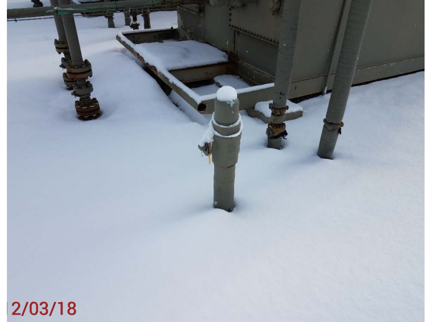
Location Photo #2, Unmarked flow line riser.
