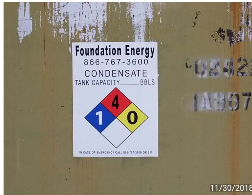
Photo 4. Tank label missing 300 bbl capacity.
