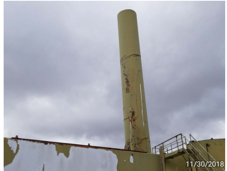
Photo 2. Missing bird protector.
