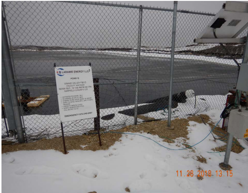
Photo #1 – Pit sign and leak detection system located on north side of pit.
