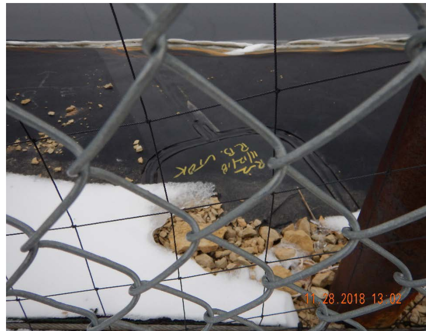
Photo #6 – Liner patch on east side of pit dated 11/12/2018.
