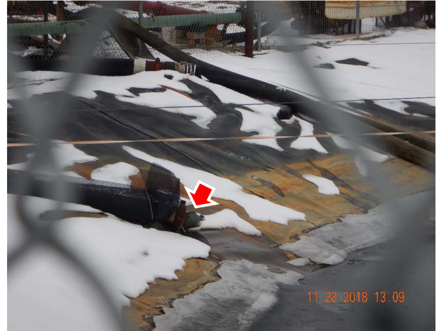
Photo #10 – Position of sandbag beneath inlet hose with hammer union located at NW corner of pit remains unaddressed from previous Field Inspection Report. Compare to Photo #11 from 11/1/2018 Field Inspection Report.
