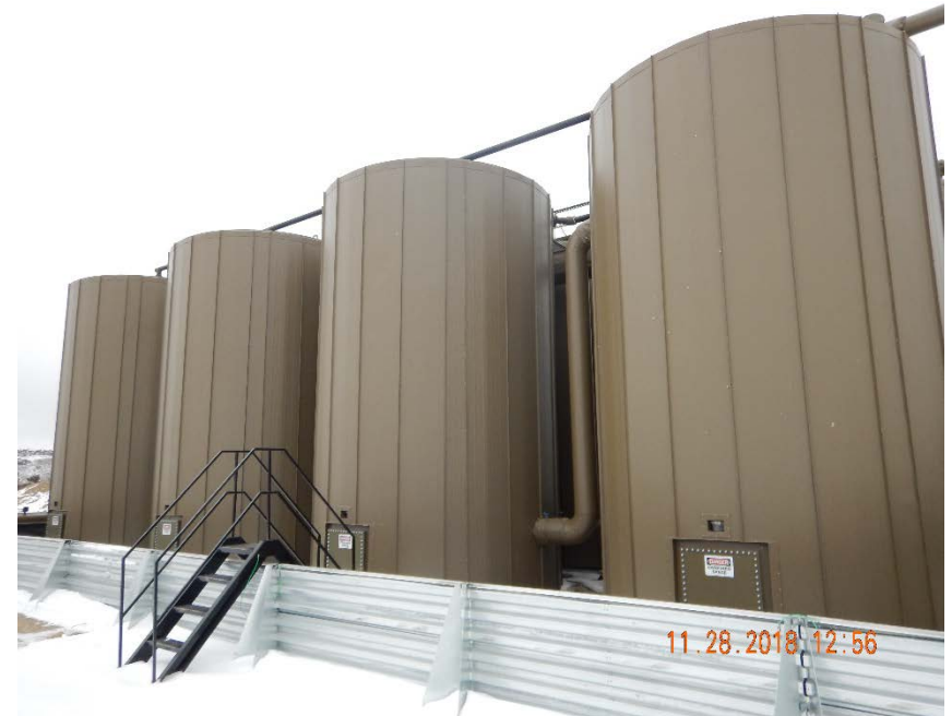
Photo #2 – Tank battery located NE of pit. Note that tanks lack content/volume labels and NFPA placards.
