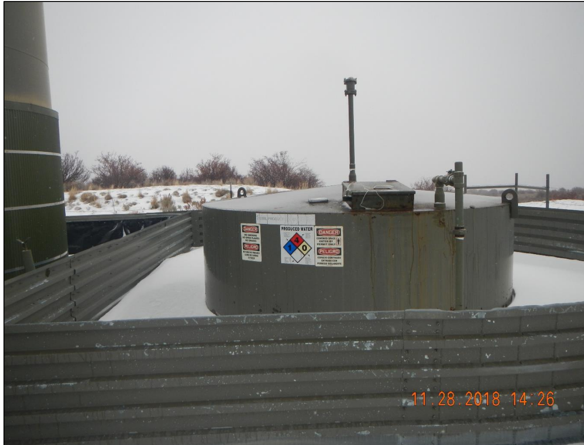
Capacity label on produced water tank is faded and cracking.
