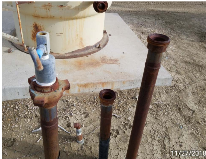
Photo 3. Uncapped or locked out tag out risers.
