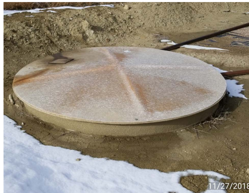
Photo 2. Buried tank without labels.
