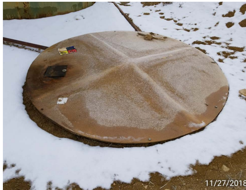
Photo 2. Buried tank without complete labeling.
