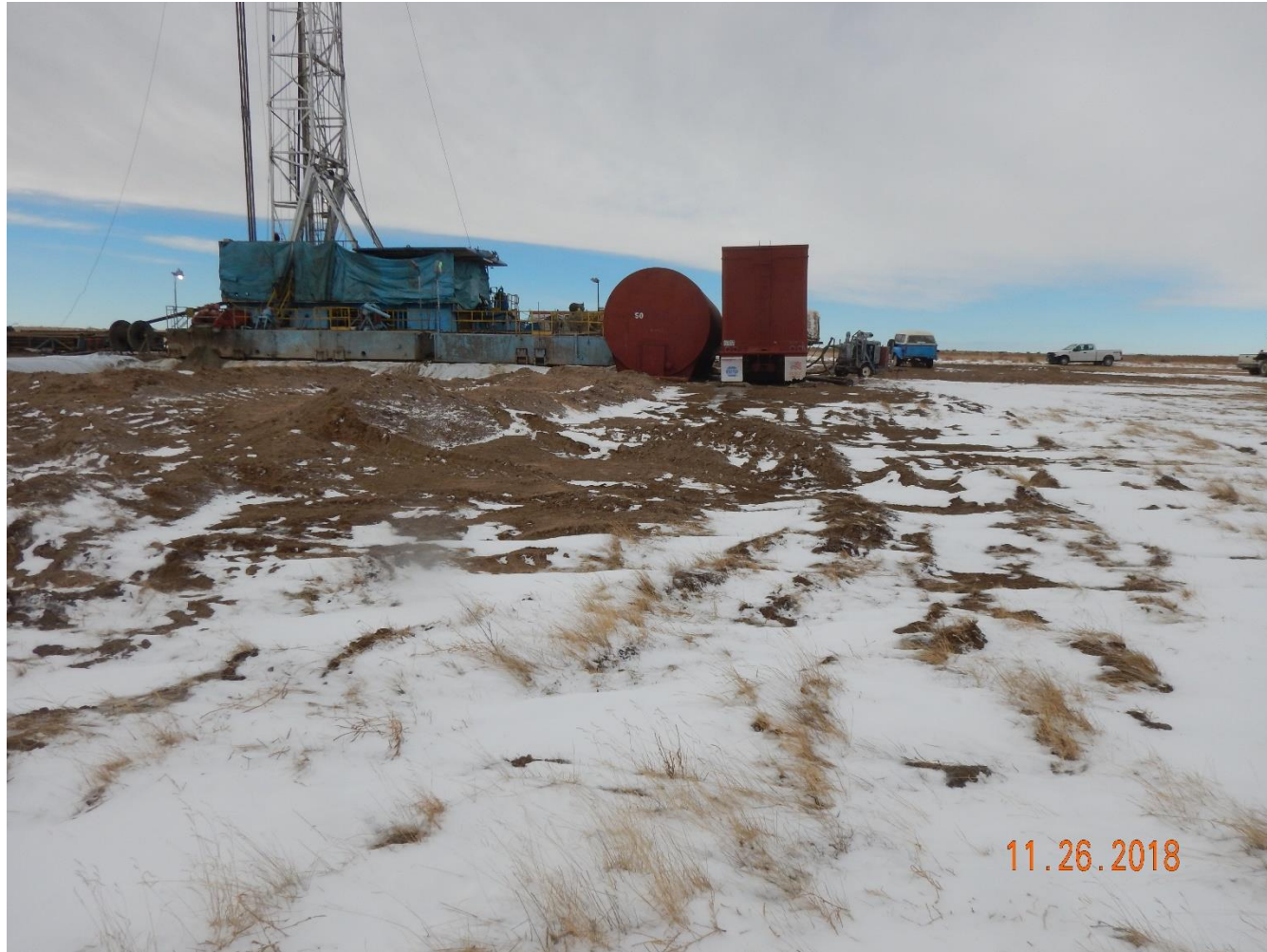
Photo 9: Photo taken from the northeast end of the pad, facing west. Operator indicated that ~3 feet of soil will be brought onto the location to build up the pad. It does not appear as though 3 feet of soils have been brought on site. Photo also shows no perimeter stormwater and erosion control BMPs have been installed on the location in accordance with 1002.f
