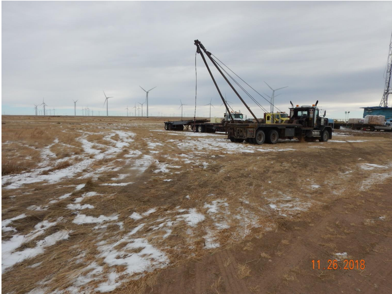
Photo 2: See comments under photo 1. Photo also shows operator appears to be storing vehicles/equipment on an area north of the pad that has not been constructed. 1002.e requires that “well sites/access roads shall be adequately sized, constructed and maintained so as to reasonably...minimize erosion, alteration of natural features, removal of surface materials and degradation due to contamination”. Location does not appear to have been constructed in such a manner to be appropriate in size to store all vehicles/equipment.
