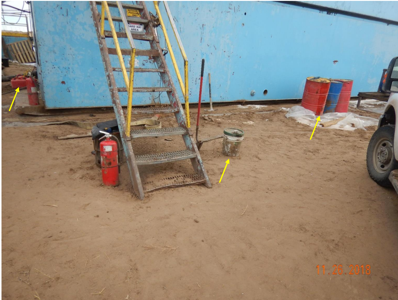
Photo 22: Photo taken from the southwest of the drill rig. Photo shows various buckets, barrels, gas cans without proper storage or secondary containment. This is improper materials management.
