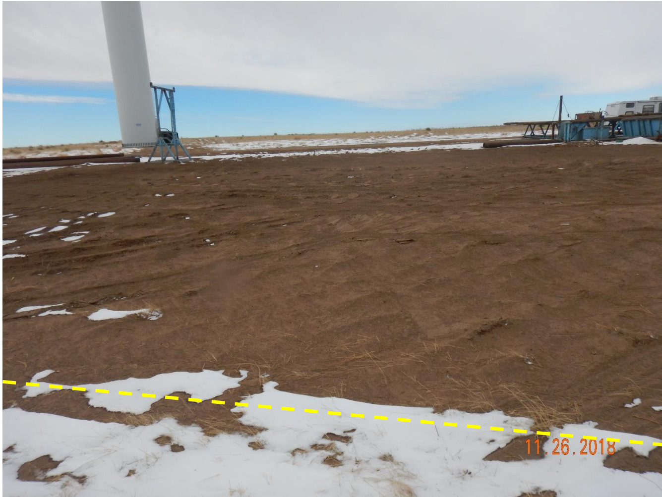
Photo 15: Photo taken from the south end of the location, facing west. Photo shows areas where soil has been brought onto the location. It does not appear as though location has been built up by 3 feet as indicated by operator. Photo shows perimeter of the pad and the adjacent lands. Photo also shows no perimeter stormwater and erosion control BMPs have been installed on the location in accordance with 1002.f
