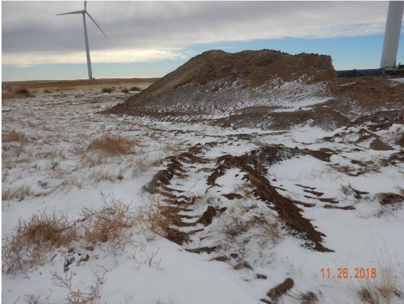
Photo 10: Photo taken from the northeast end of the pad, facing west. Photo shows soil excavated from the pit. 2A states pit to be 8 feet deep. Photo shows topsoil and subsoils do not appear to have been separated and stored or marked/documented. It appears that topsoil and subsoil horizons have all been placed into one soil stockpile. Photo also shows no perimeter stormwater and erosion control BMPs have been installed on the location in accordance with 1002.f
