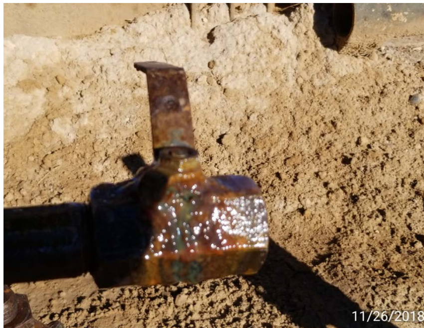
Photo 3. Wellhead valve leaking gas at handle.
