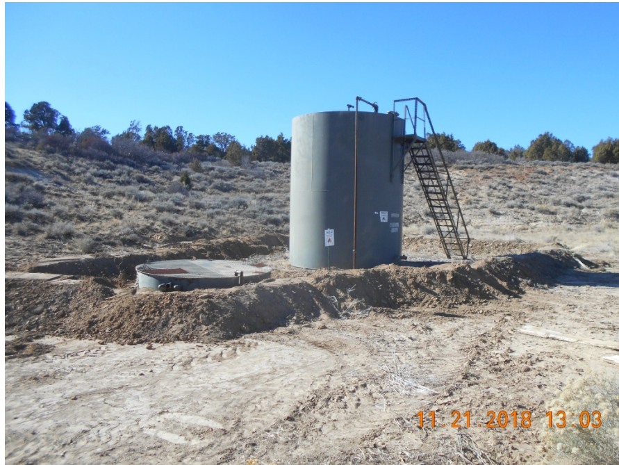
Tank battery. Berms repaired. CA completed
