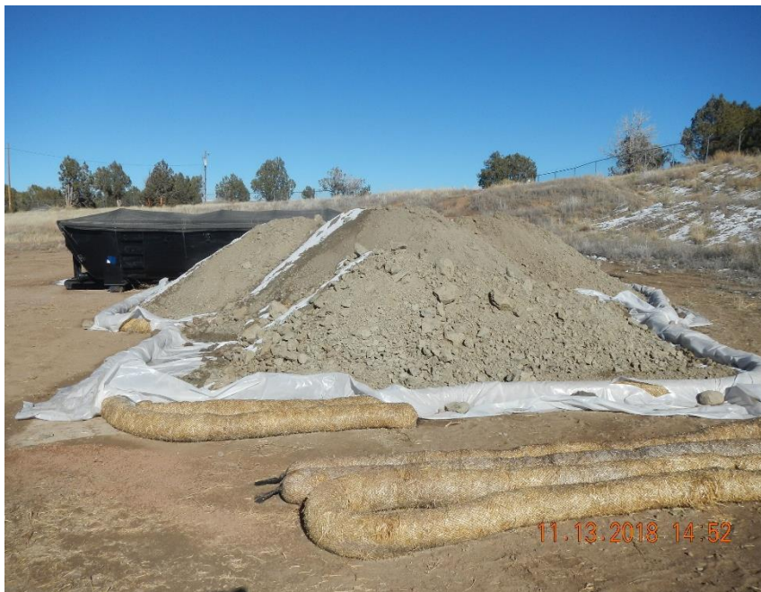
Excavated material staged on Thomas Jacquez E #1 location with liner.
