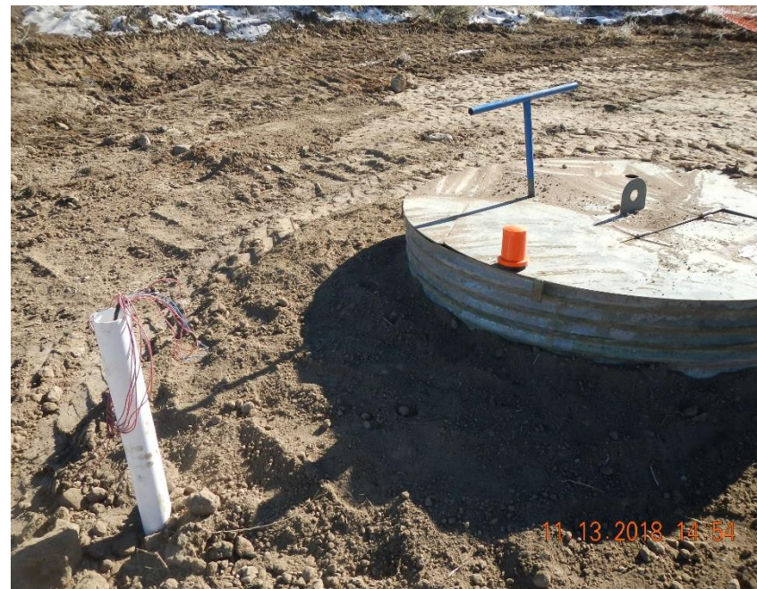
Valve can replaced after repairs to pipeline were completed.
