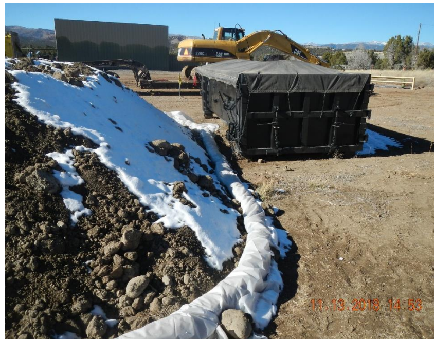
Soil dumpster and temporary stock pile of excavated material.
