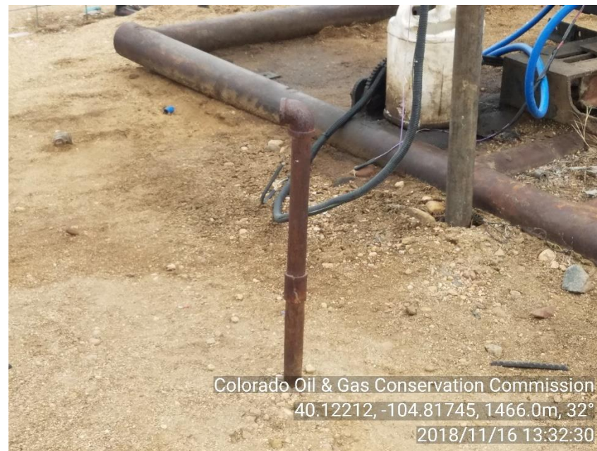
PHOTO 4: UNMARKED UNUSED RISER
