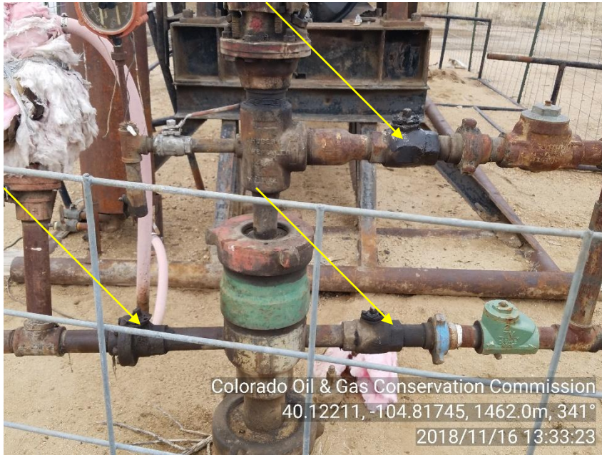
PHOTO 7: VALVES LEAKING
