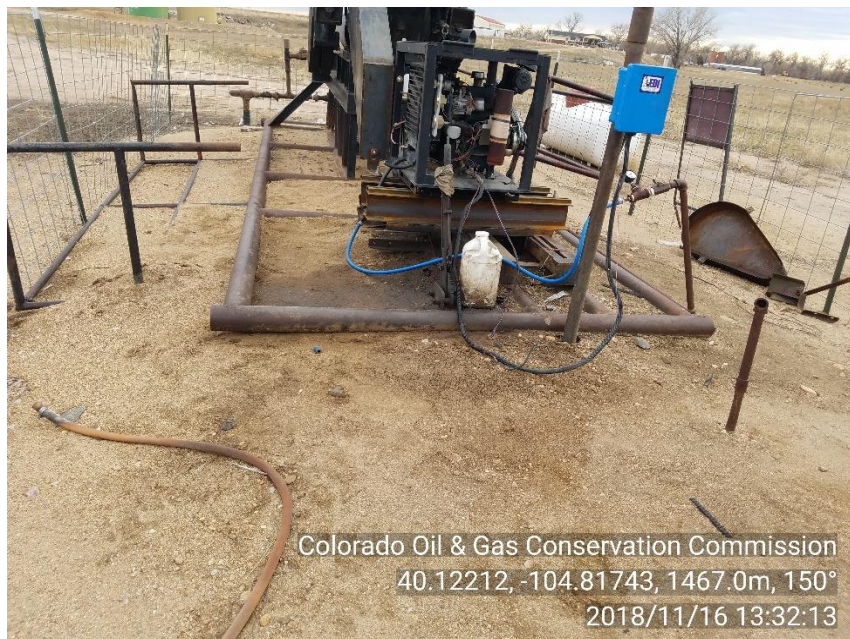
PHOTO 3: STAINED SOIL UNDER PRIME MOVER
