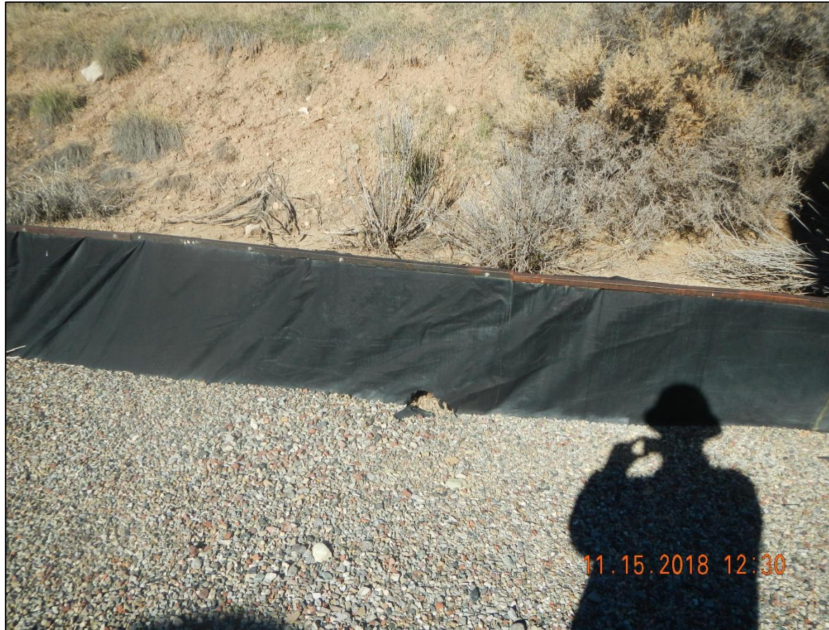
Hole in tank berm liner.
