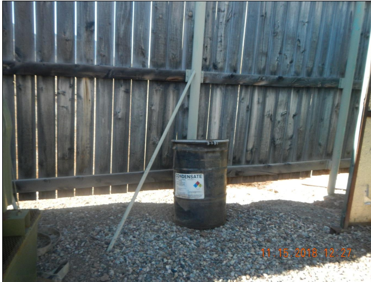
Barrel of condensate at compressor with out secondary containment.
