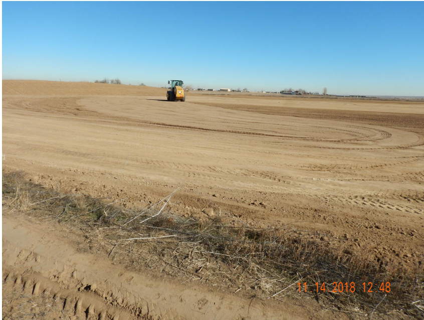
Photo 5. Photo taken from the western perimeter of the location, facing East. Operator in-process of stabilizing the pad with road base.
