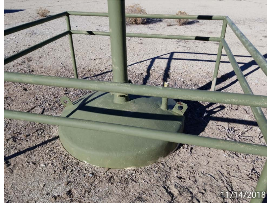
Photo 2. Tank without labeling and berm.
