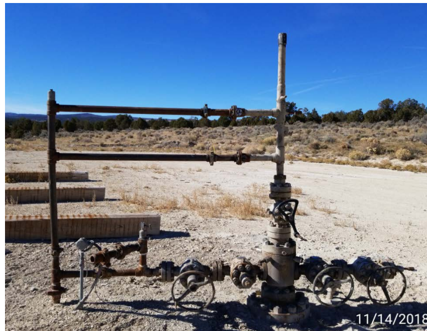
Photo 2. Wellhead flow lines are connected.
