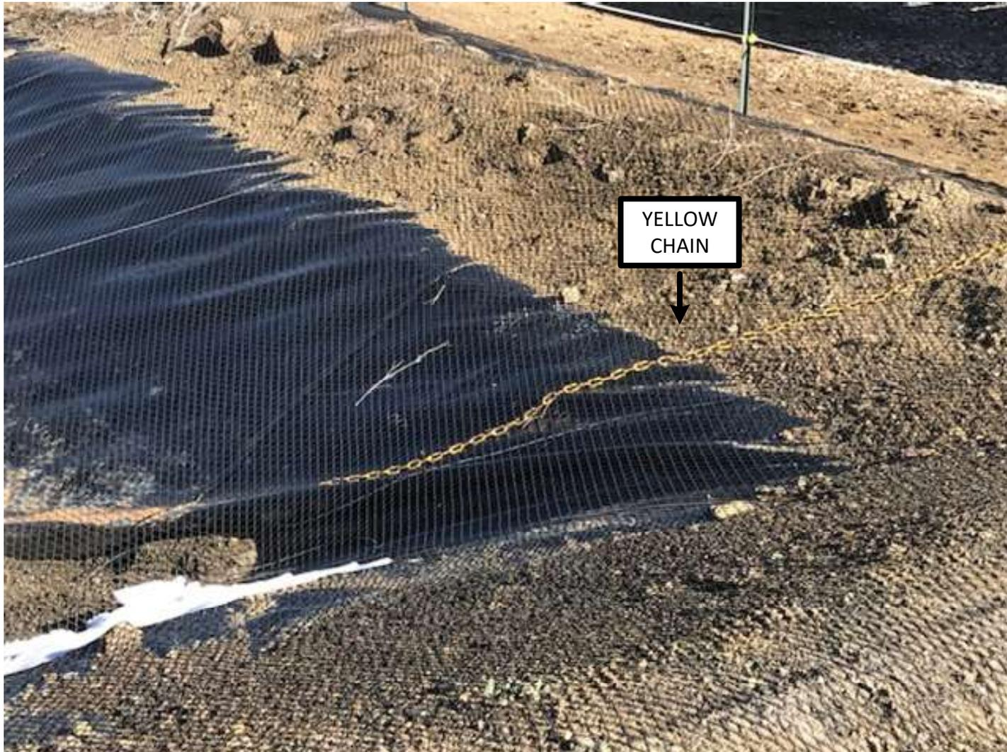
A YELLOW CHAIN WAS INSTALLED IN THE PRODUCTION PIT TO MONITOR (2) FOOT OF FREEBOARD BETWEEN THE TOP OF THE PIT WALL AND THE FLUID LEVEL OF THE PIT.
