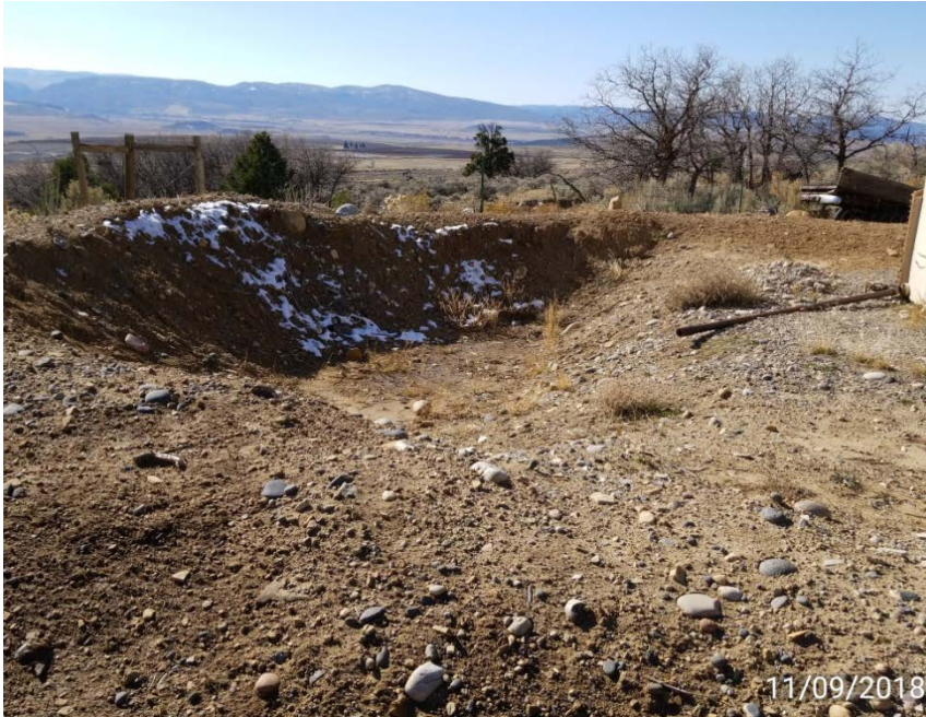
Photo 5. Pit in inside tank berm.
