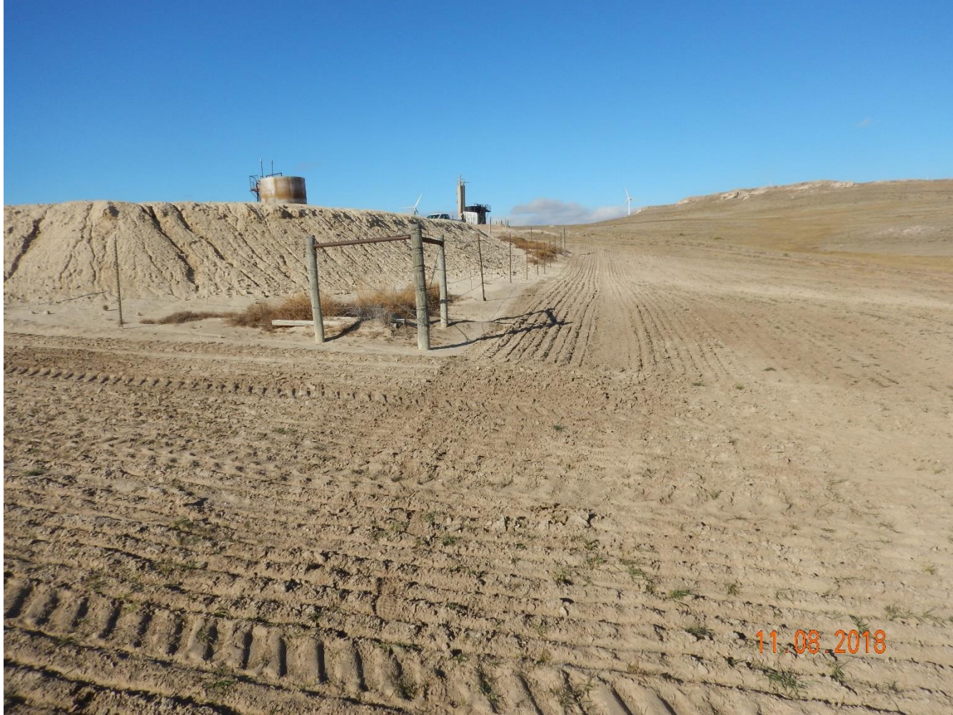
Photo 6: Photo taken from the southeast end of the pit, facing north. Photo shows additional reclamation activities appear to have been conducted on the spill areas to the south of the pit. Photo also shows that no sediment, erosion or stabilization controls have been installed.
