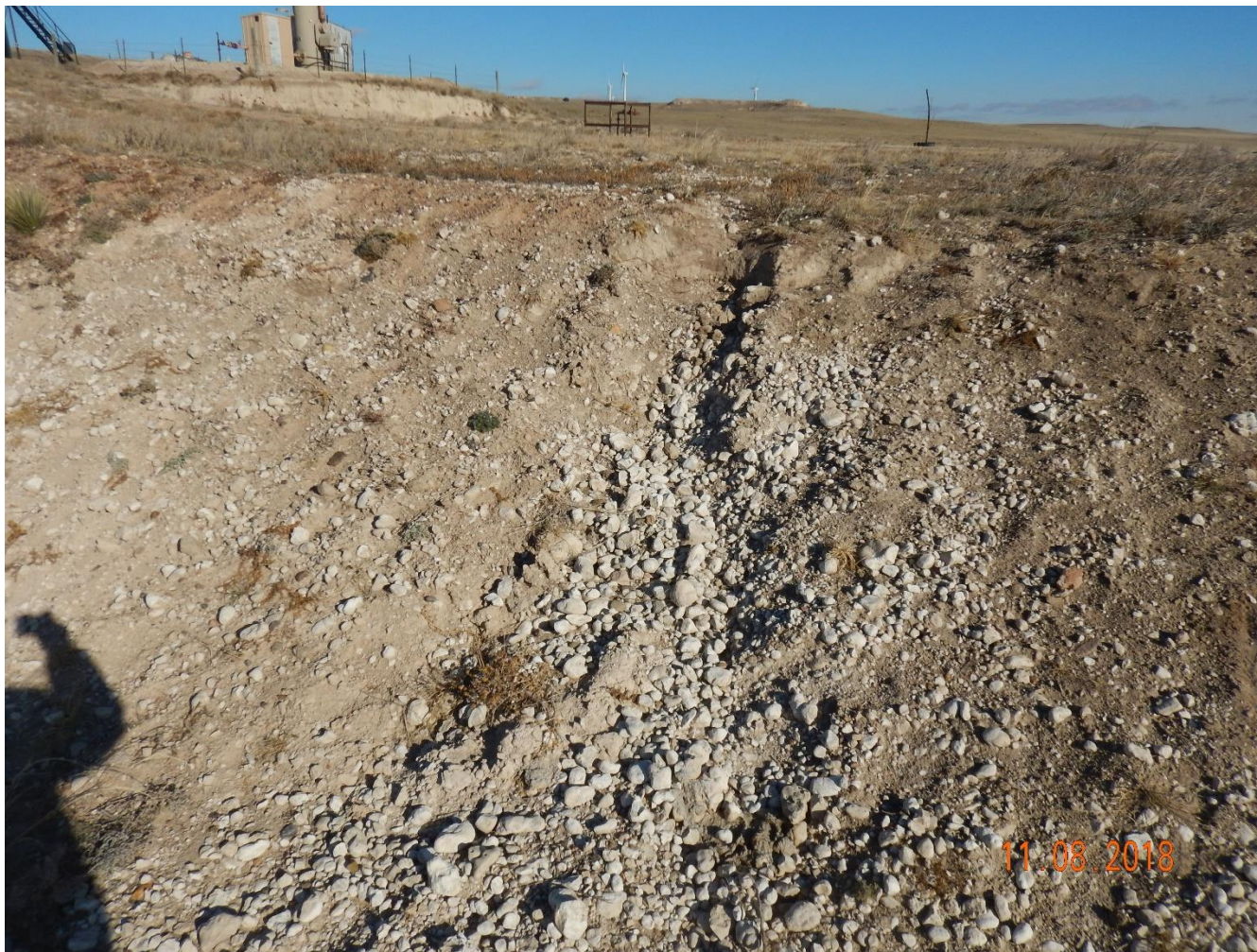
Photo 12: Photo taken from the west end of the location, facing east. Photo shows gully erosion due to stormwater runoff from the pad. Photo shows erosion has not been repaired and no BMPs have been installed to mitigate degradation.
