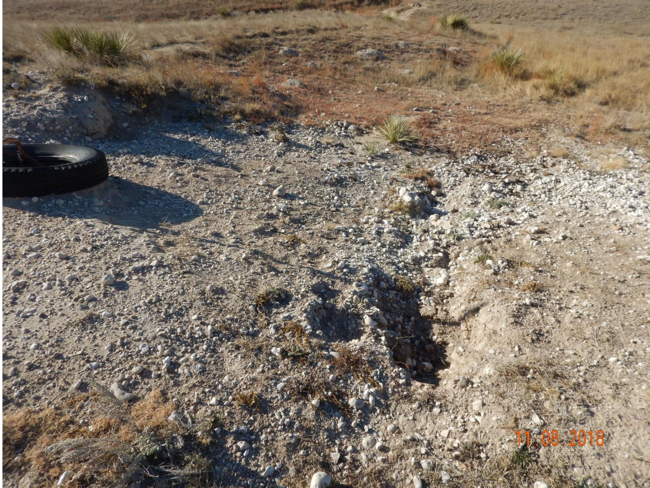
Photo 10: Photo taken from the west end of the location, facing west. Photo shows gully erosion due to stormwater runoff from the pad. Photo shows erosion has not been repaired and no BMPs have been installed to mitigate degradation.
