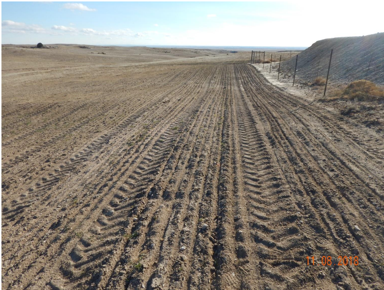
Photo 3: Photo taken from the east end of the pit, facing south. Photo shows additional reclamation activities appear to have been conducted on the spill areas to the south of the pit. Photo also shows that no sediment, erosion or stabilization controls have been installed.
