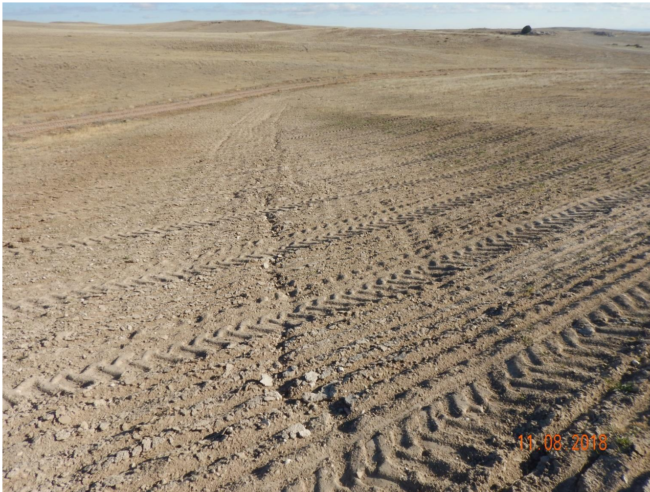
Photo 4: Photo taken from the east end of the pit, facing east. Though additional reclamation activities appear to have been conducted, no sediment, erosion or stabilization controls have been installed, allowing for stormwater erosion degradation to recur.
