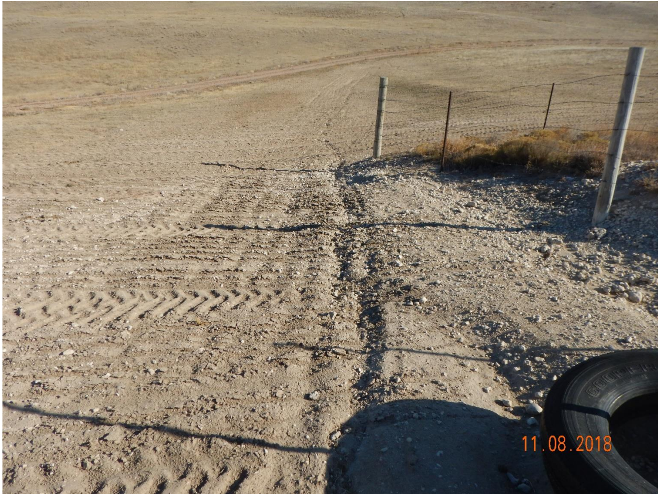
Photo 2: Photo taken from the east end of the pad, facing east. Though additional reclamation activities appear to have been conducted, no sediment, erosion or stabilization controls have been installed, allowing for stormwater erosion degradation to recur.
