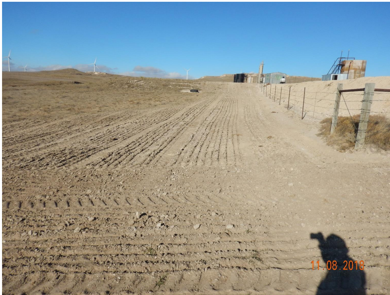
Photo 9: Photo taken from the southwest end of the pit, facing north. Photo shows additional reclamation activities appear to have been conducted on the spill areas to the south of the pit. Photo also shows that no sediment, erosion or stabilization controls have been installed.
