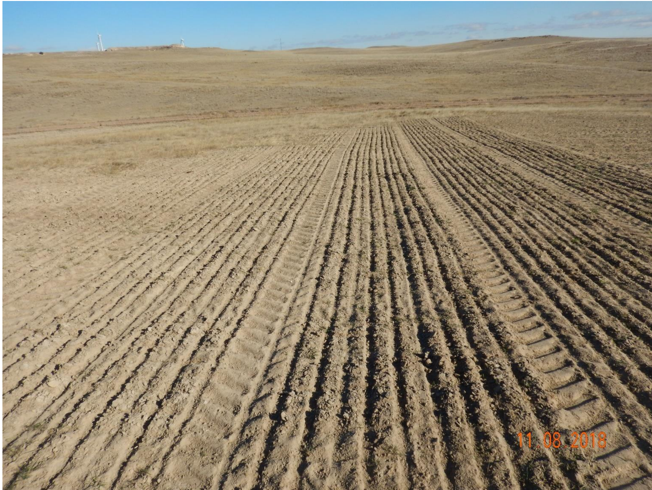
Photo 5: Photo taken from the southeast end of the pit, facing east. Photo shows additional reclamation activities appear to have been conducted on the spill areas to the south of the pit. However, areas appear to have been seeded up/down the slope rather than parallel to the contour. This may likely contribute to future erosion concerns as the furrows have created a straight path that will allow stormwater to concentrate and accelerate downslope. Photo also shows that no sediment, erosion or stabilization controls have been installed.
