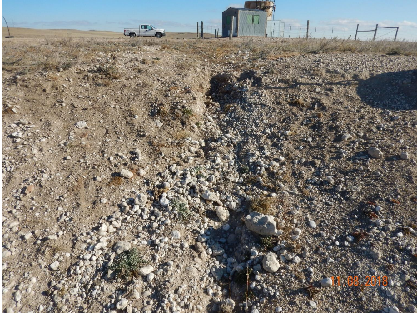
Photo 11: Photo taken from the west end of the location, facing east. Photo shows gully erosion due to stormwater runoff from the pad. Photo shows erosion has not been repaired and no BMPs have been installed to mitigate degradation.
