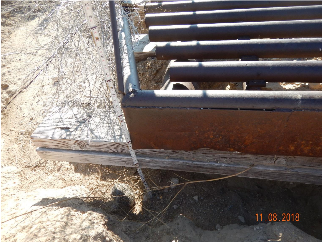
Photo 2: Photo taken from the access road. Photo shows erosion degradation occurring at the cattle guard has not been repaired. Photo also shows ~ 2 feet of soil has been washed out beneath the cattle guard.
