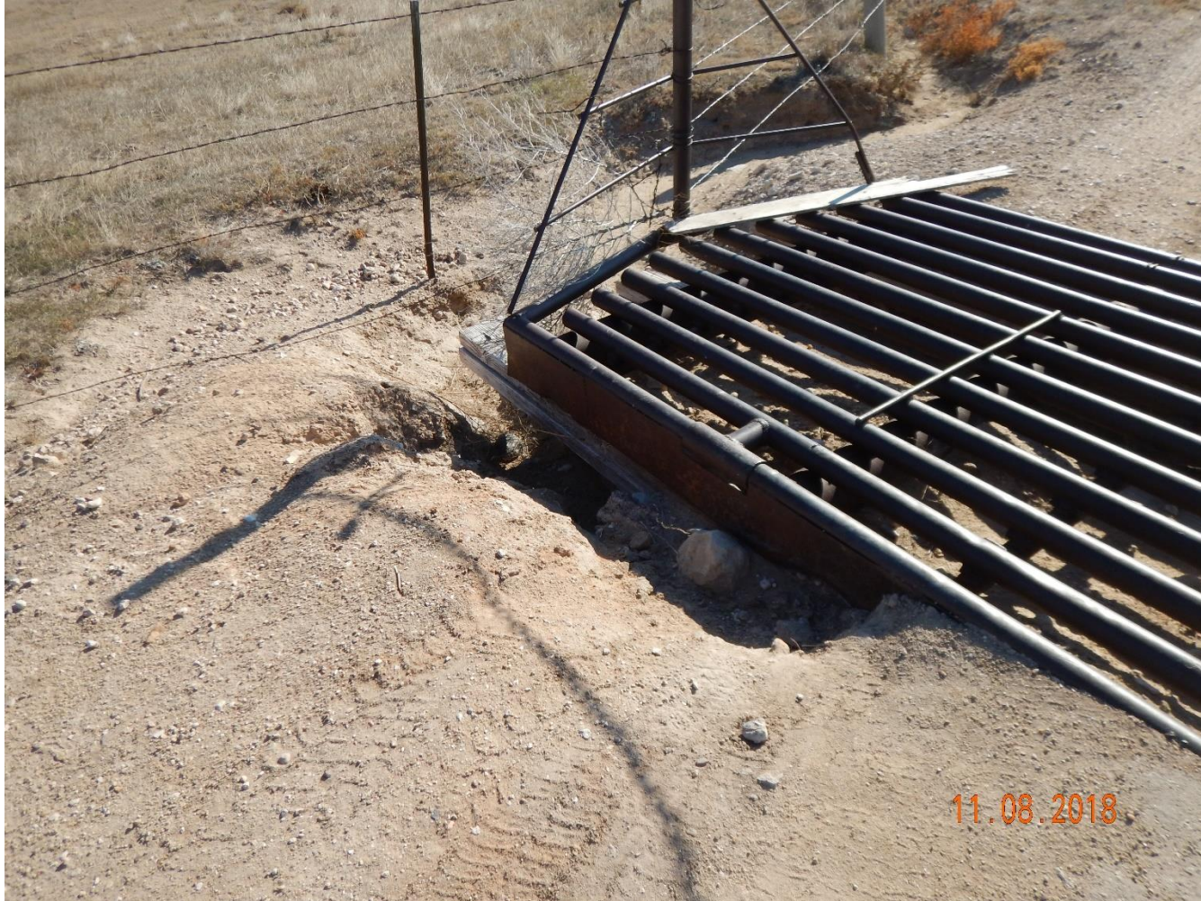
Photo 1: Photo taken from the access road. Photo shows erosion degradation occurring at the cattle guard has not been repaired.
