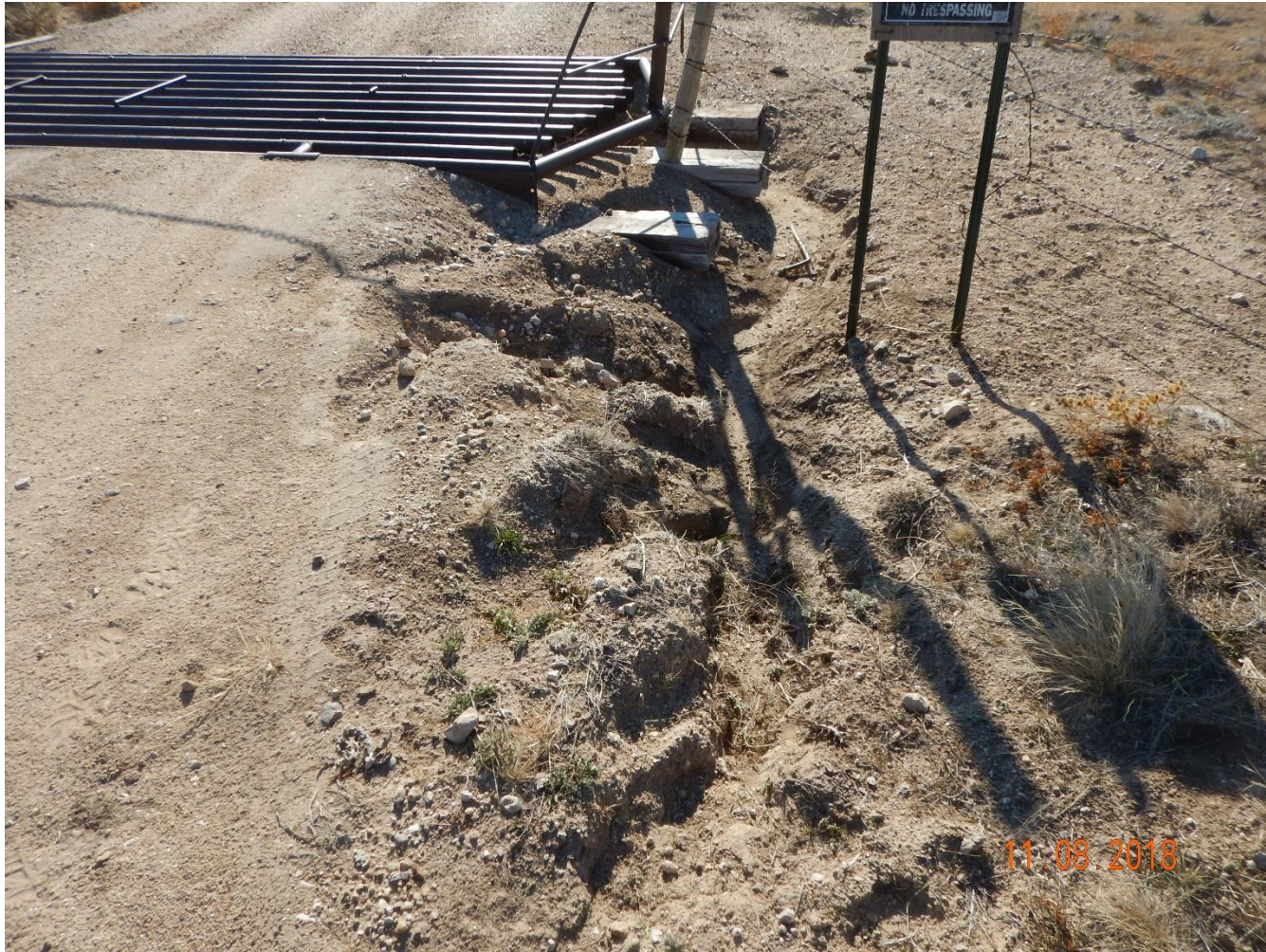
Photo 3: Photo taken from the access road. Photo shows erosion degradation occurring at the cattle guard has not been repaired.
