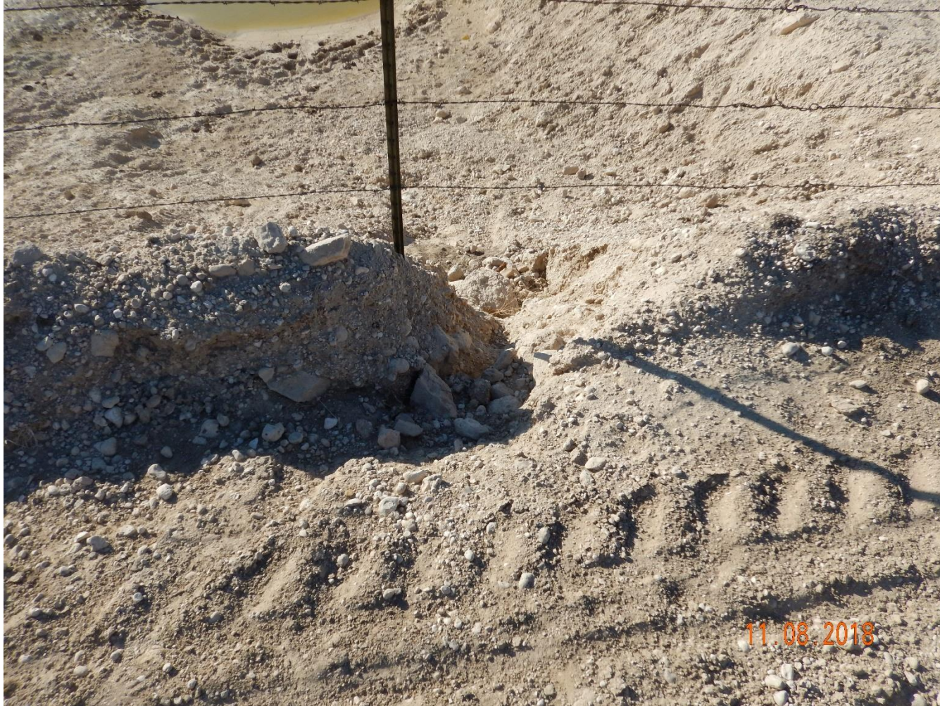
Photo 5: Photo taken from the west end of the pad (east end of pit). Photo shows gully erosion from the pit has not been addressed.
