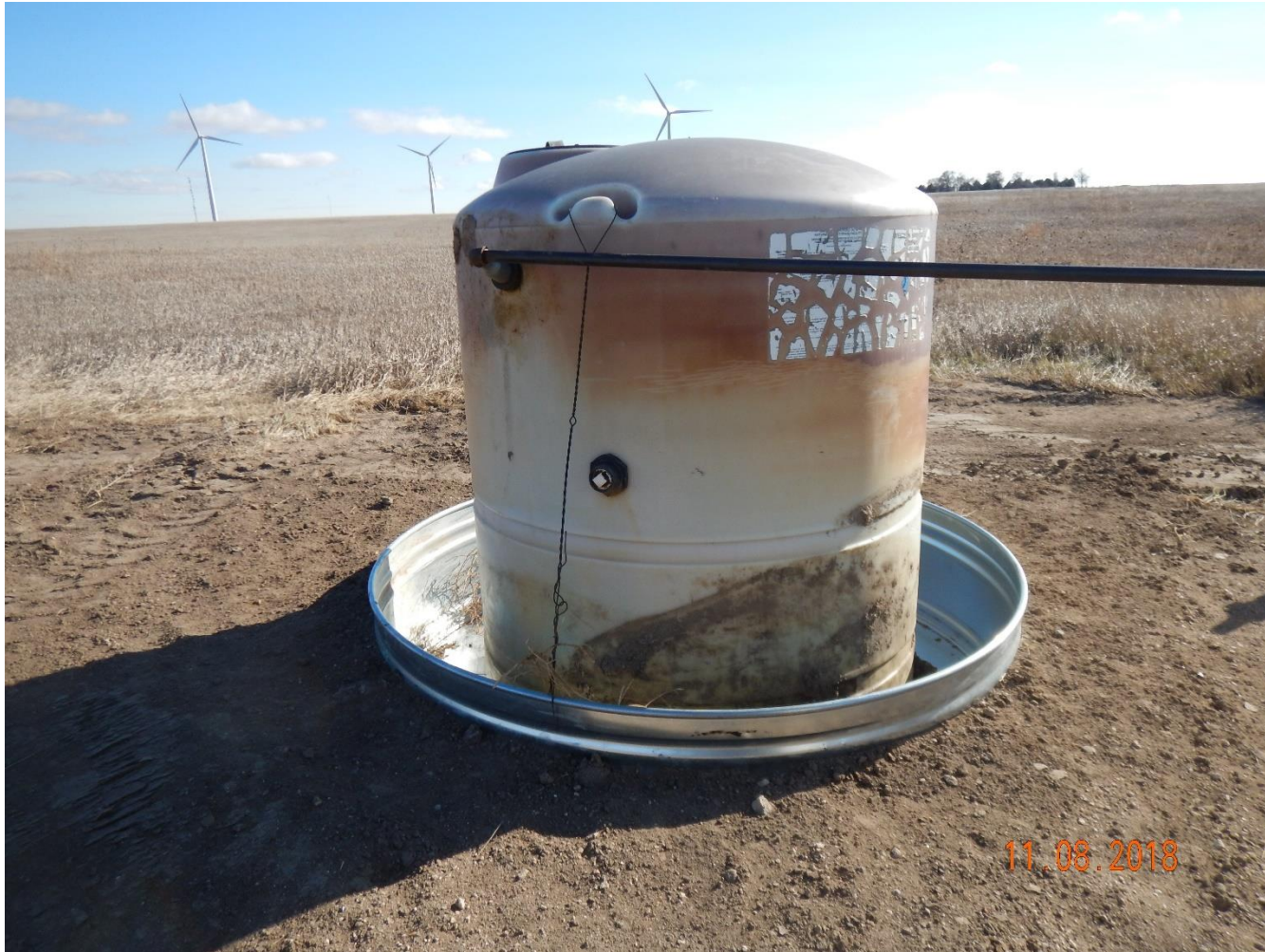
Photo 3: Photo taken from meter shed, facing south. Previous inspection required plastic tank to be placed back. Operator appears to have installed secondary containment and returned the tank. Previous inspection also required operator to replace signage/placards on tank. Photo shows signage/placards have not been replaced.
