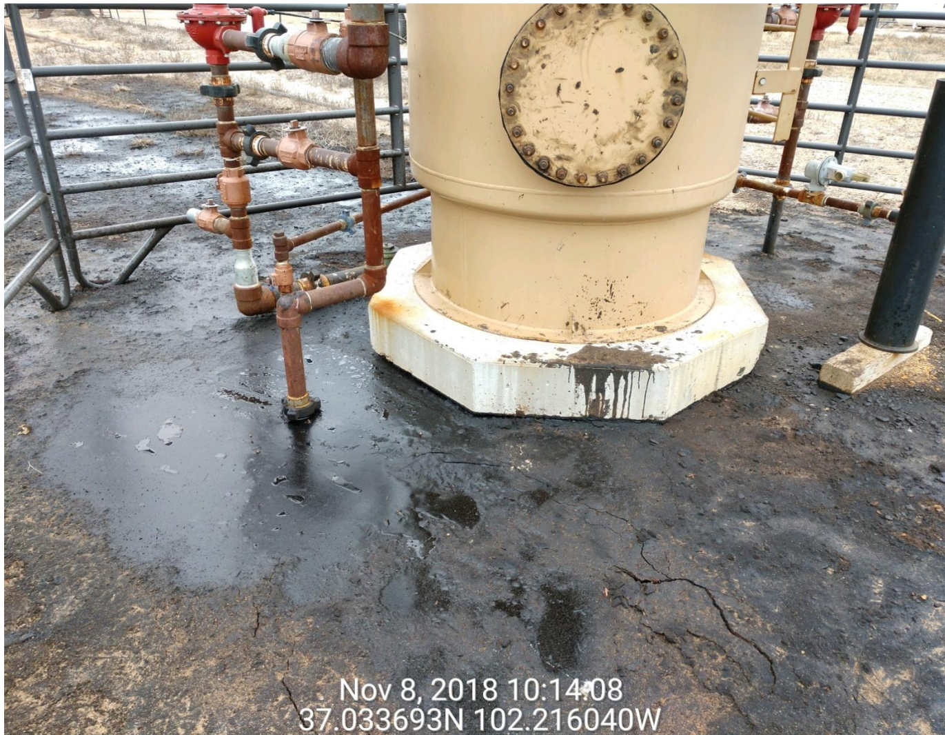
Spill around heater treater
