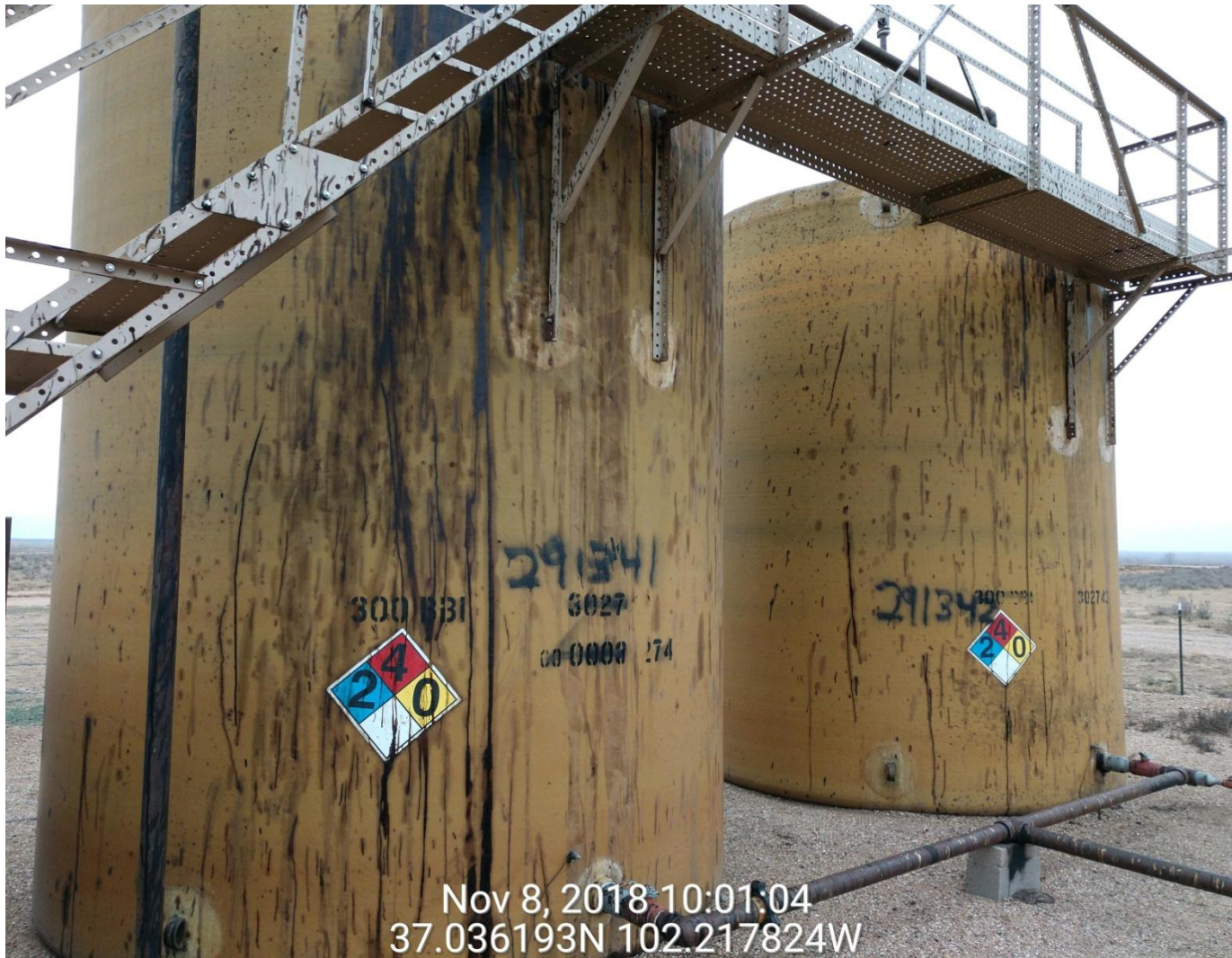
Tanks missing labels. Visible signs of tank overflow.
