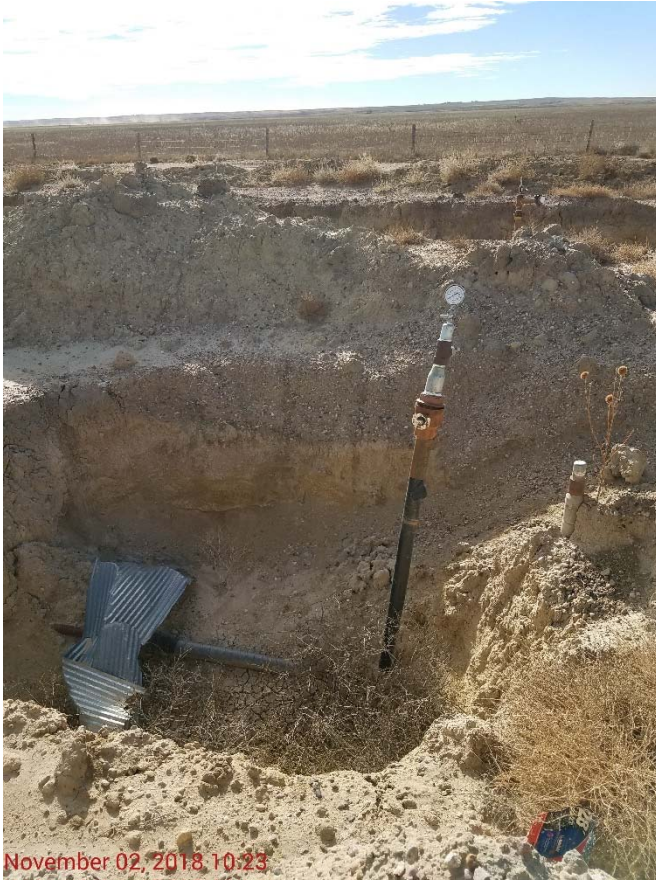
Photo 3 – Produced water injection line, near former injection building and adjacent former tank battery.
