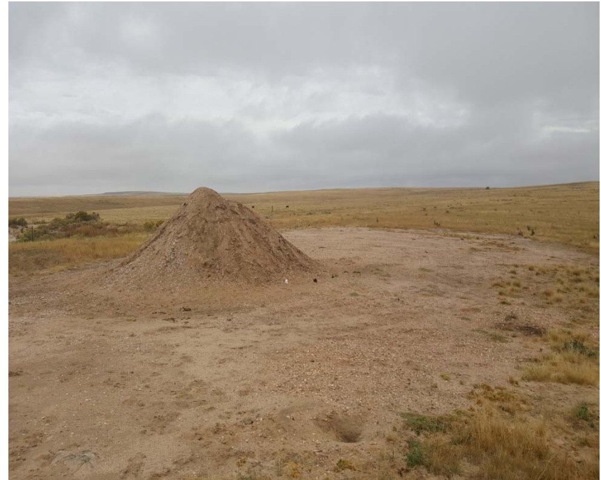
Photo #8 Stockpile of dirt mixed with gravel on former battery location. Some small localized areas of oil staining in disturbed areas.
