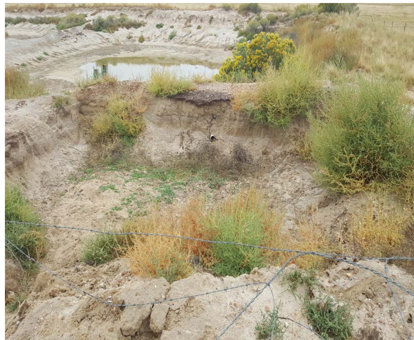
Photo #6 Former skim pit (Fac ID #109707) excavation looking west. Oily waste along top of west wall.
