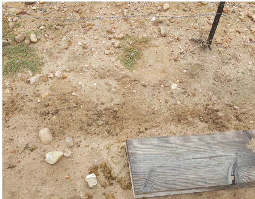
Photo #2 Localized oil stained soil at pumping unit.
