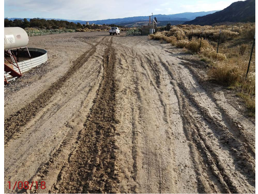
Location Photo #4, Access road storm water issue unresolved.
