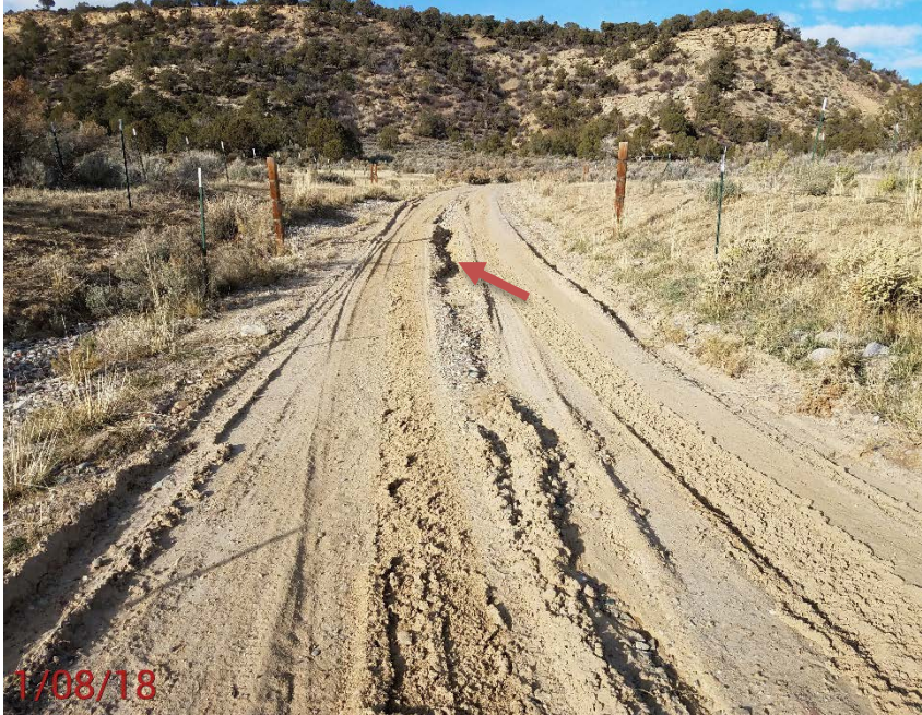
Location Photo #5, Sediment being moved onto location. Rilling occurring in middle of road.
