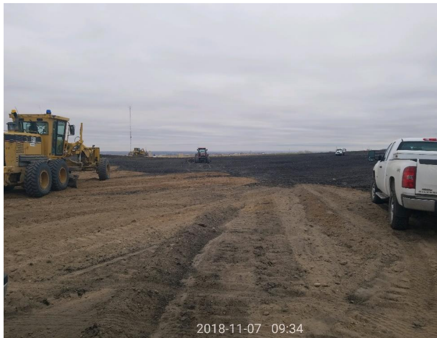
Photo 1 – Equipment on site deep ripping location.
