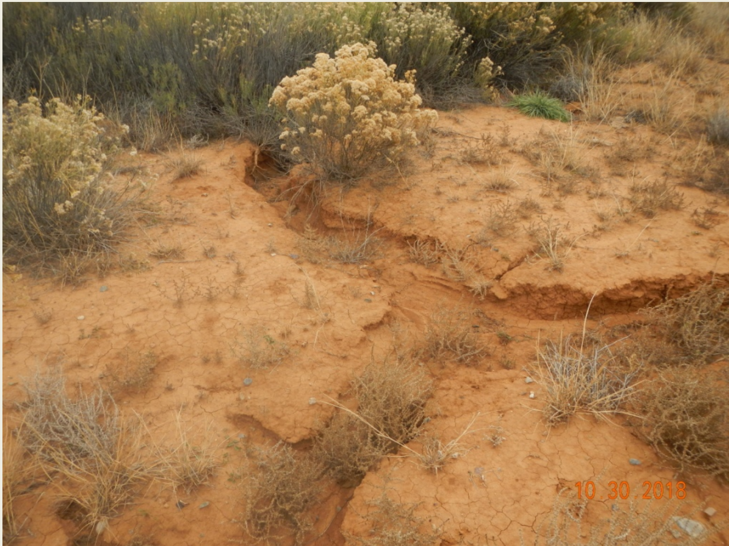
Photo 6. View of erosional channel within the northern file slope, approximately 2.5 feet wide and deep>
