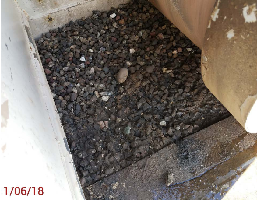
Location Photo #7, Oily stained rock under separator by burner unit.
