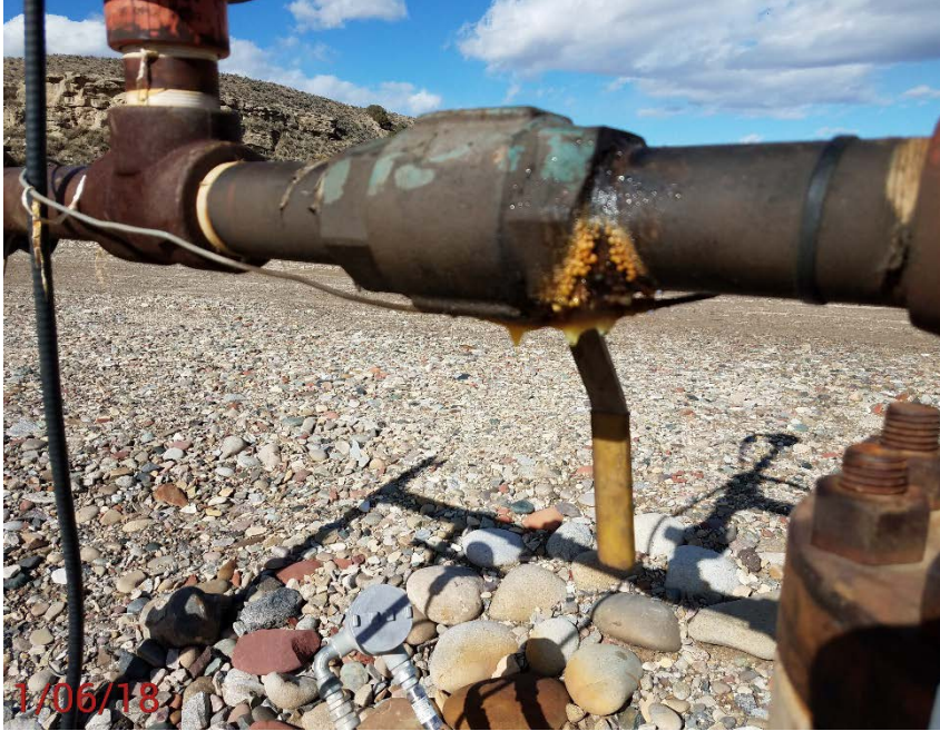
Location Photo #9, Mechanical condition of valves in flow line.
