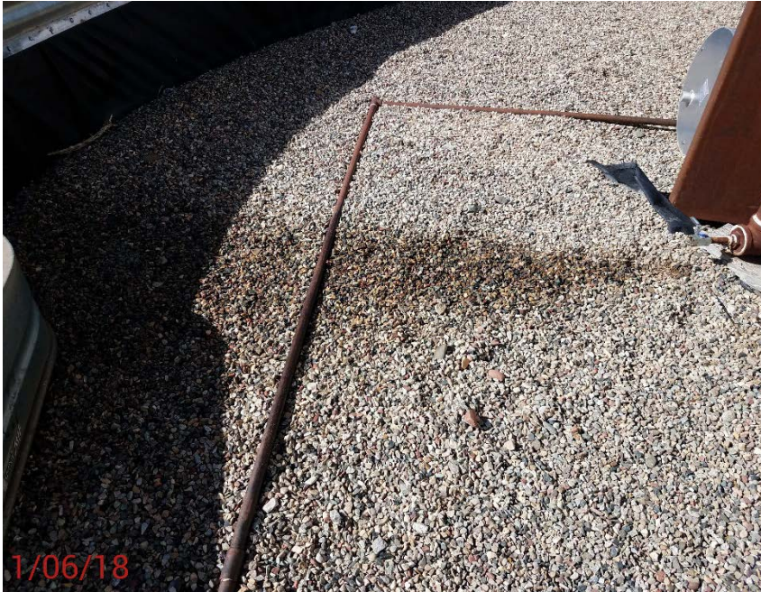
Location Photo #3, Oil stained rock in battery containment.
