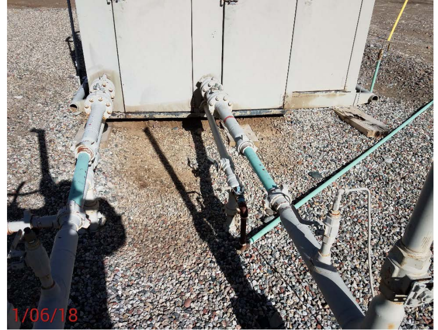
Location Photo #6, Stained rock under and around separator.
