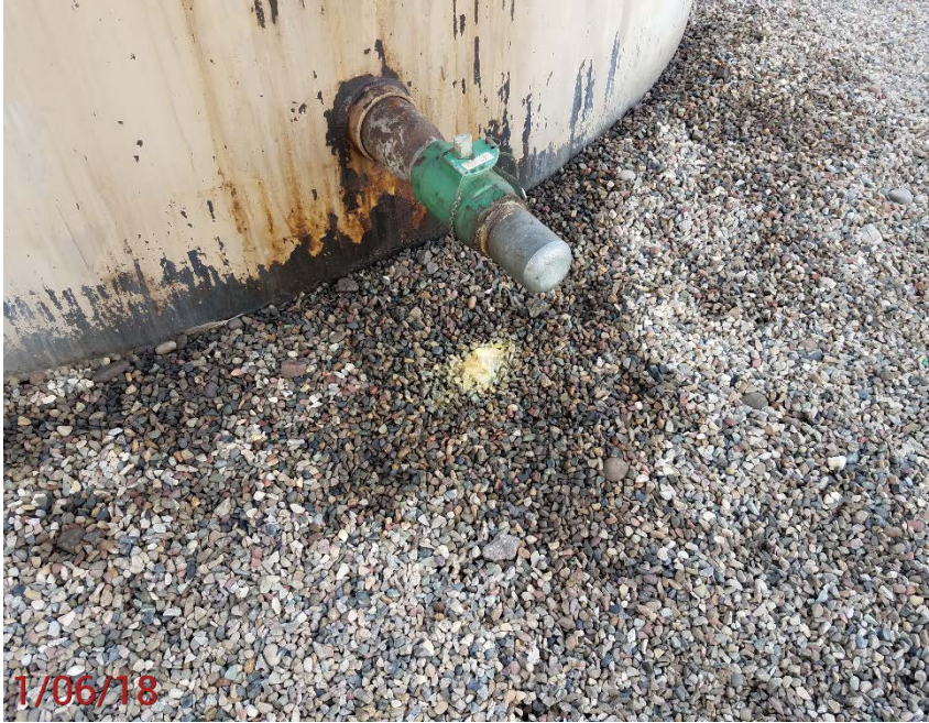
Location Photo #5, Oil stained rock in battery containment. Mechanical condition of valves.
