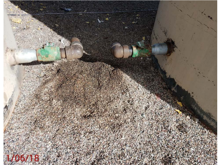
Location Photo #2, oil stained rock in battery containment.
