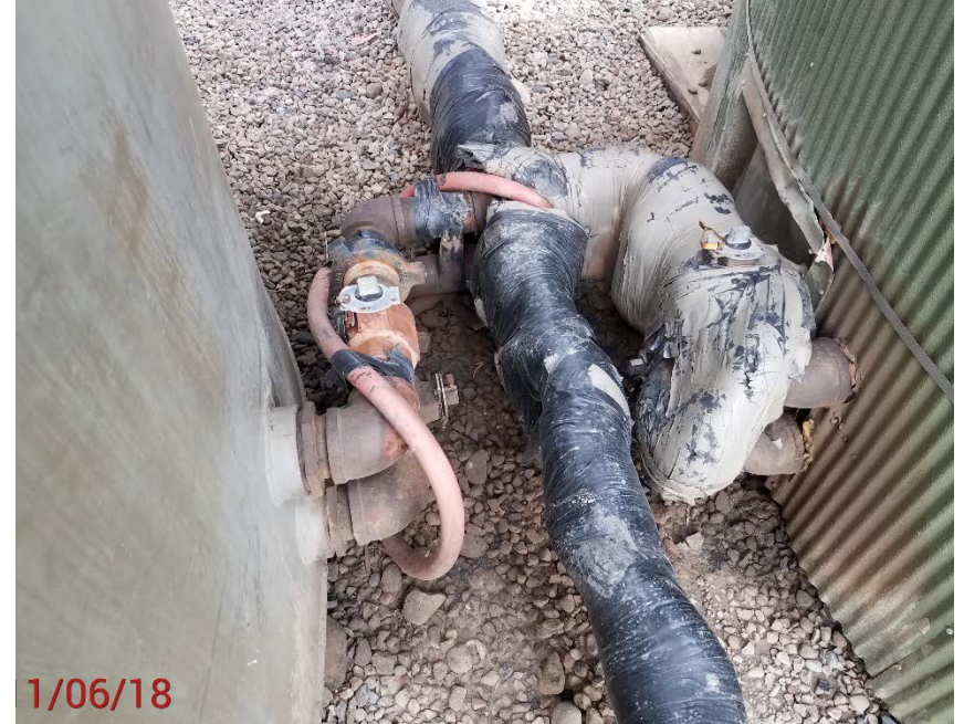
Location Photo #4, Stained rock below valves.
