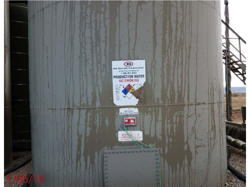
Location Photo #6, Missing BBL capacity, Inaccurate sign, Non legible.
