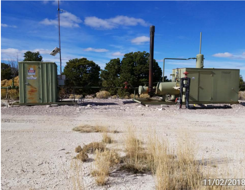
Gas meter building and separator
