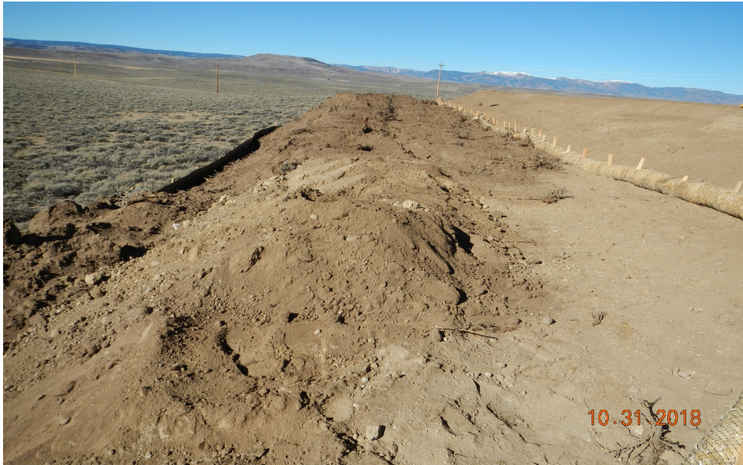
Photo#1: Topsoil has been segregated and protected.
