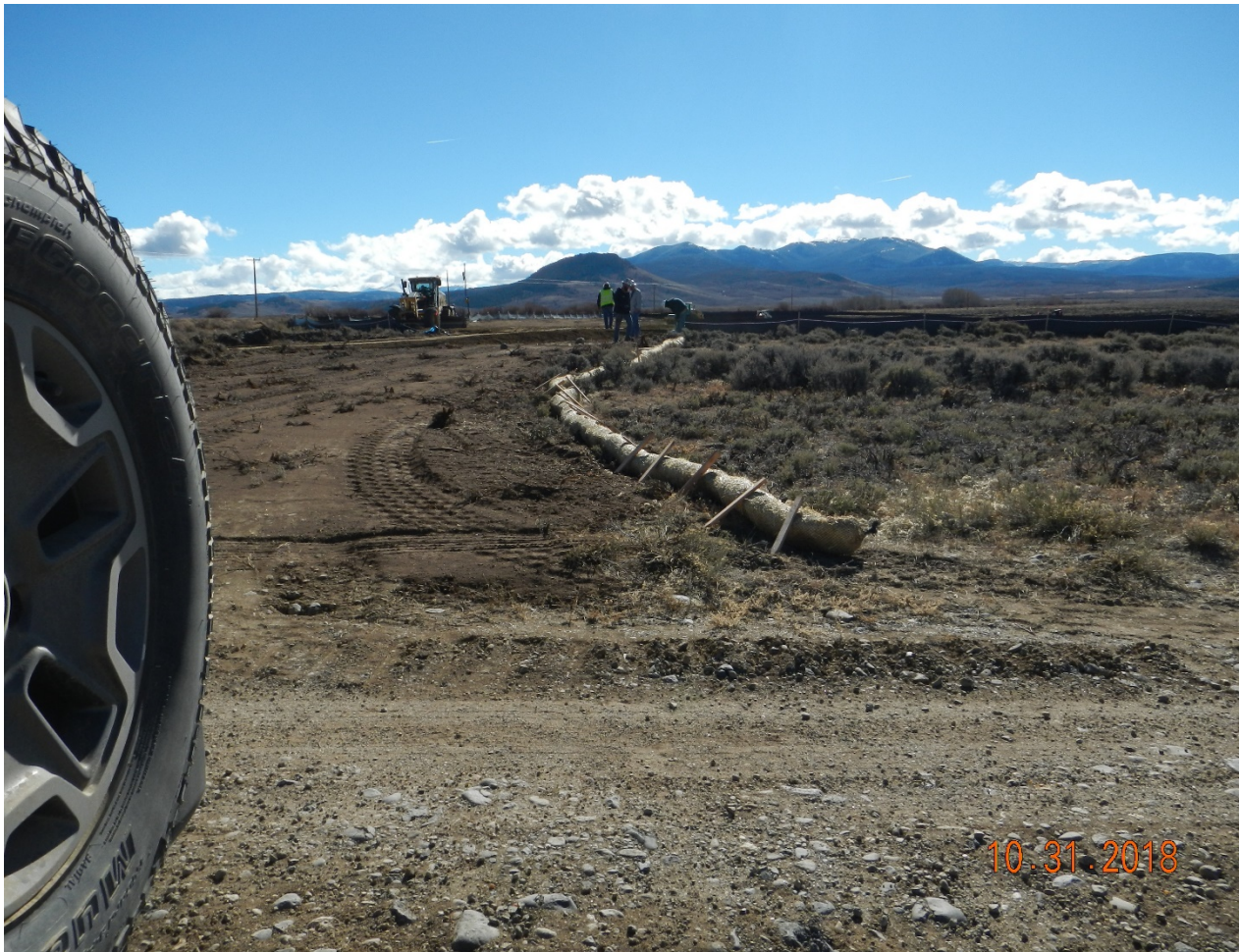
Photo#3: Bmp repairs & installations were in progress.
