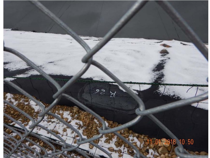
Photo #4 – Additional patch observed in liner on east side of pit. Liner has been repaired in response to previous Field Inspection Report (doc #681701069).
