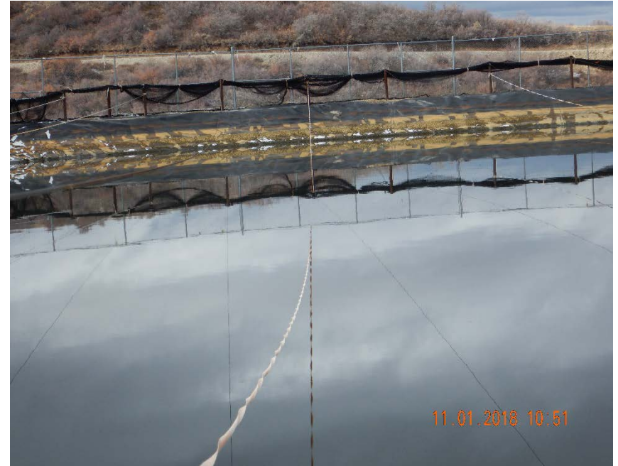
Photo #6 – Ratchet strap on south end of pit sagging into pit contents.
