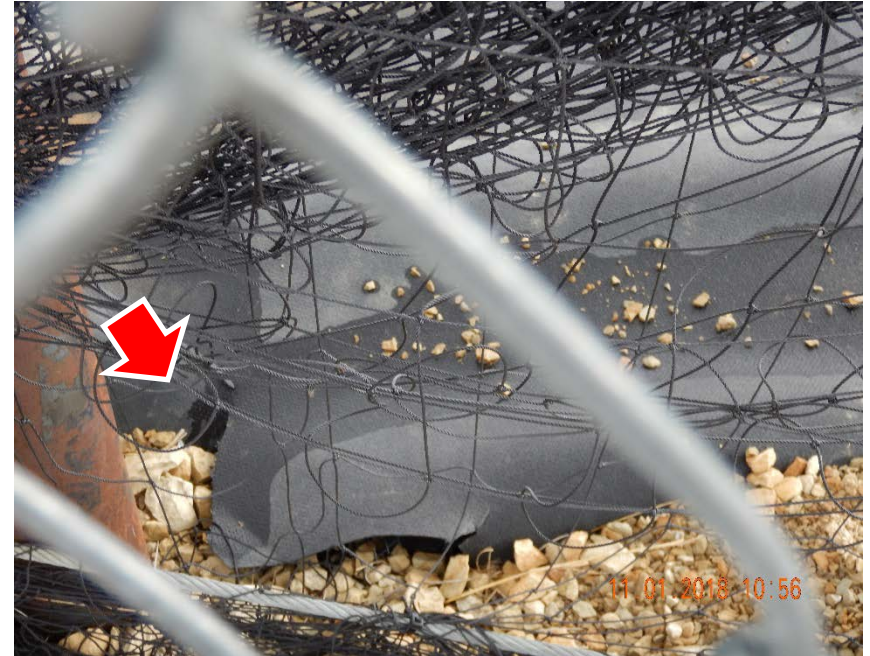
Photo #14 – Tear in pit liner observed in SW corner of pit, along anchor trench.
