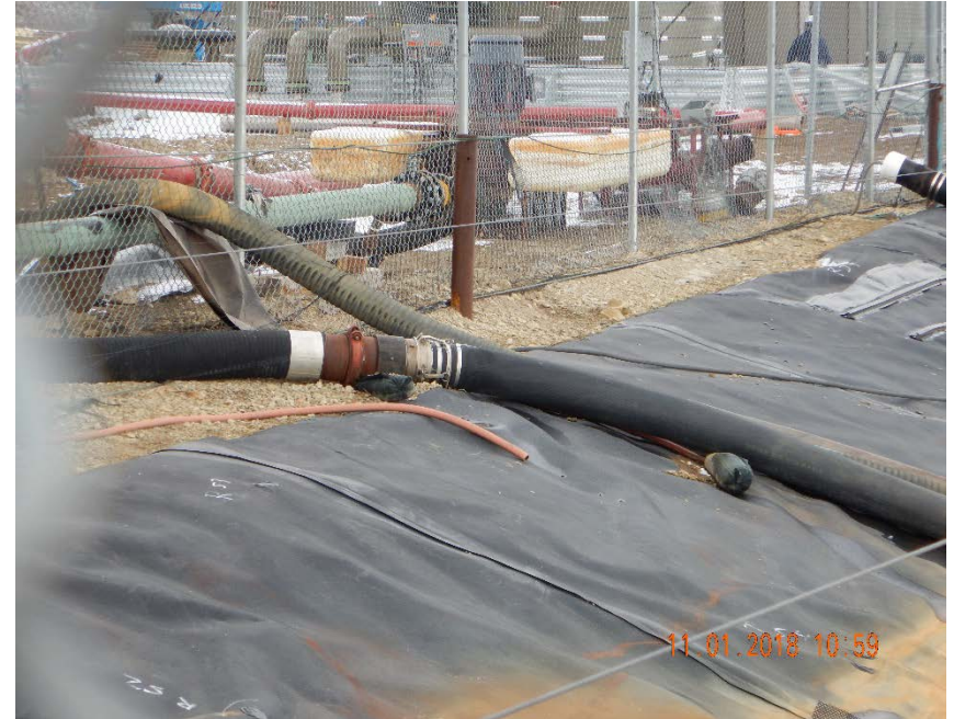
Photo #12 – Second inlet hose in NW corner of pit has been repositioned to prevent direct contact between metal fittings and pit liner.
