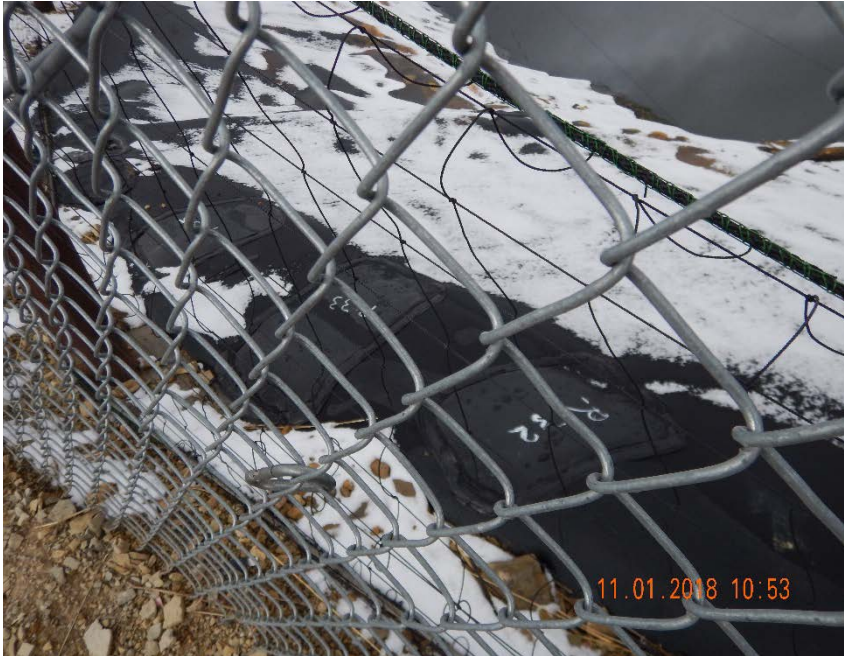
Photo #5 – Patches observed in SE corner of pit liner. Liner has been repaired in response to previous Field Inspection Report (doc #681701069).
