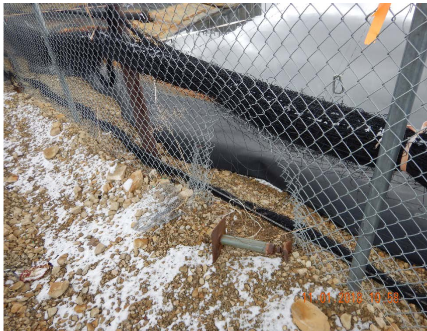
Photo #9 – Hole in NW corner of pit fence.
