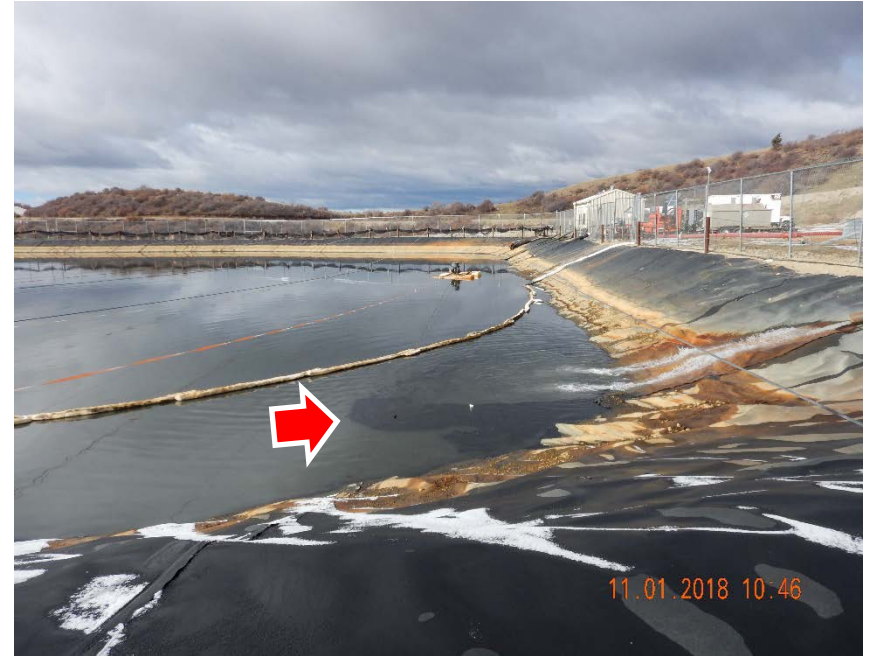
Photo #2 – View of north side of pit from NE corner. Note that bird netting was absent from pit and free product was present on top of pit fluids in NE corner (red arrow). Operator was notified about oil on pit via phone on inspection date.
