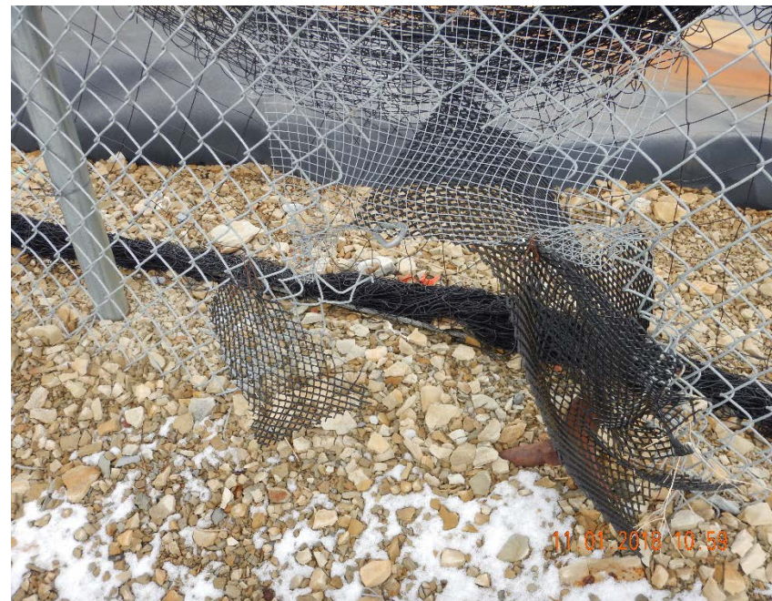
Photo #10 – Additional hole in NW corner of pit fence.
