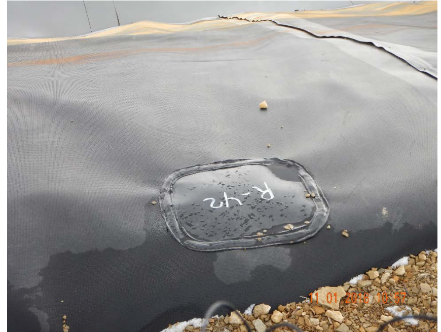
Photo #8 – Additional patch observed in liner on west side of pit.
