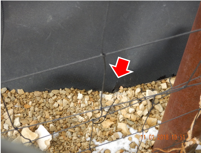
Photo #13 – Tear in pit liner observed in SE corner of pit, along anchor trench.
