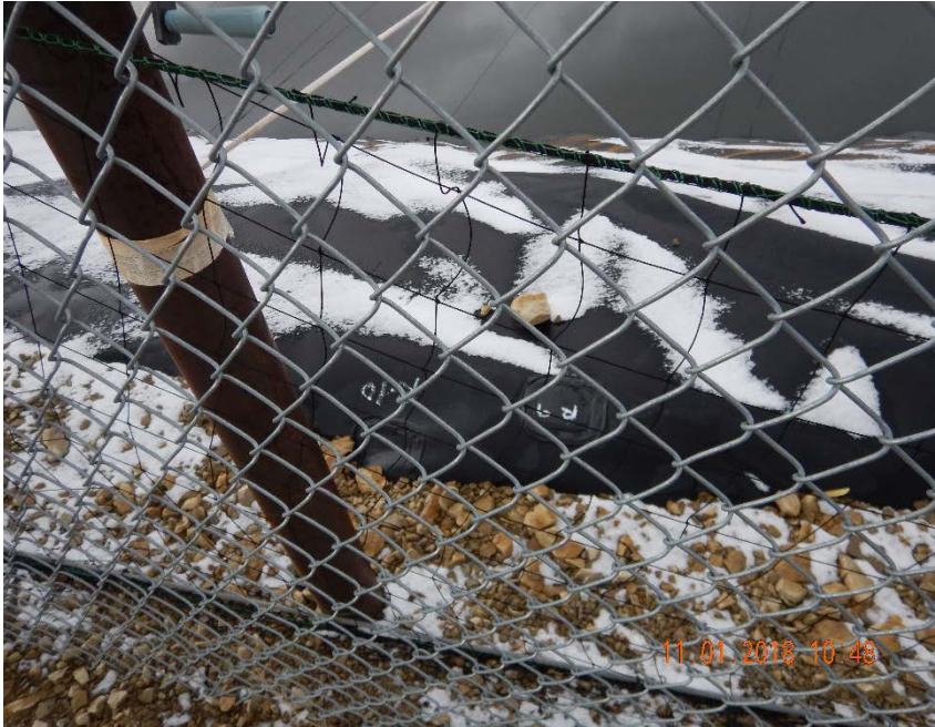
Photo #3 – Patches observed in liner on east side of pit. Liner has been repaired in response to previous Field Inspection Report (doc #681701069).
