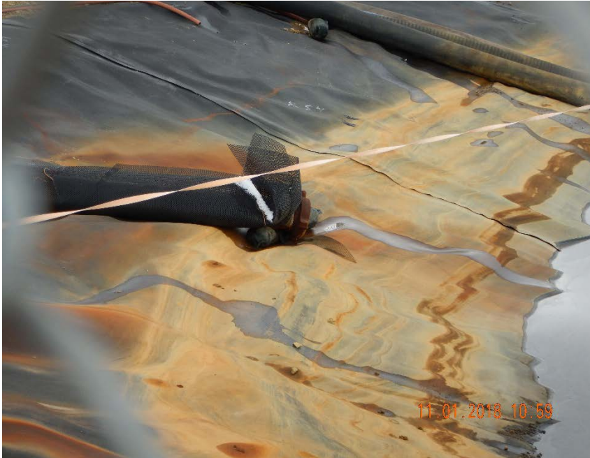
Photo #11 – Sandbag beneath inlet hose in NW corner of pit has been repositioned to prevent direct contact between hammer union and pit liner.
