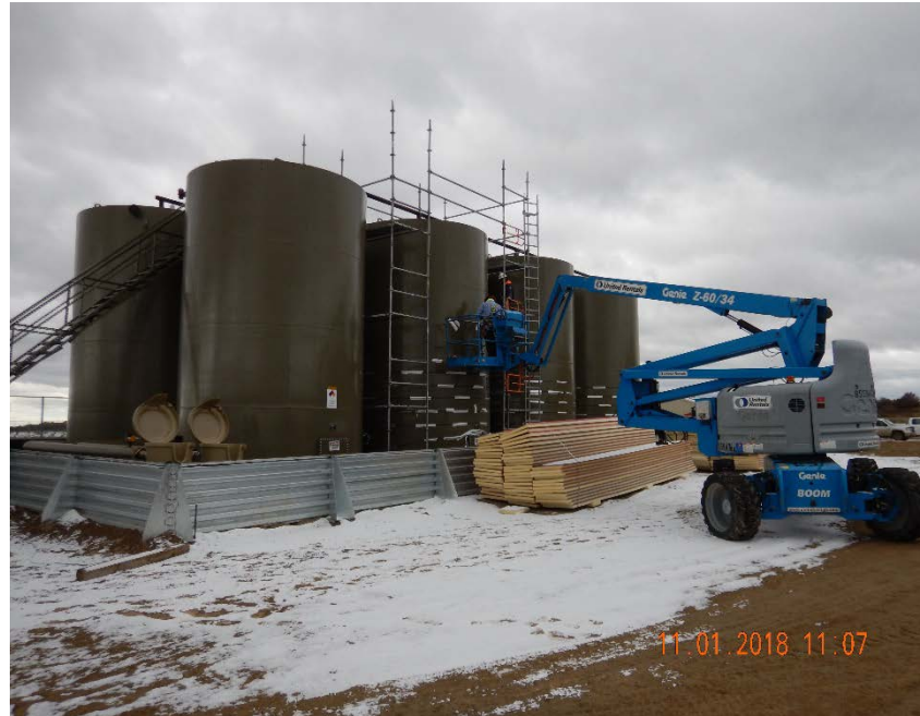
Photo #15 – Contractors were on location to install tank insulation on inspection date.
