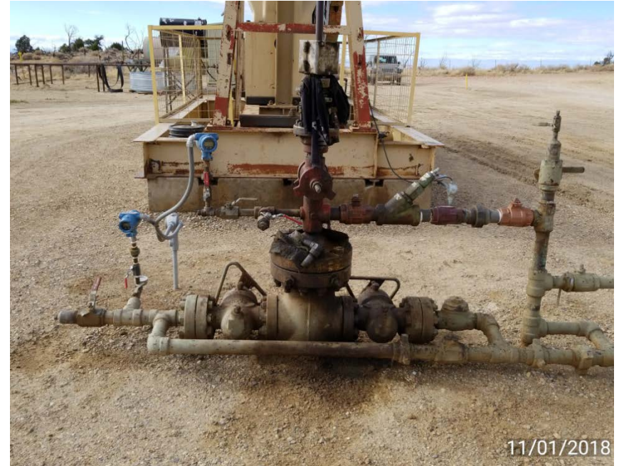
Oil on ground at wellhead
