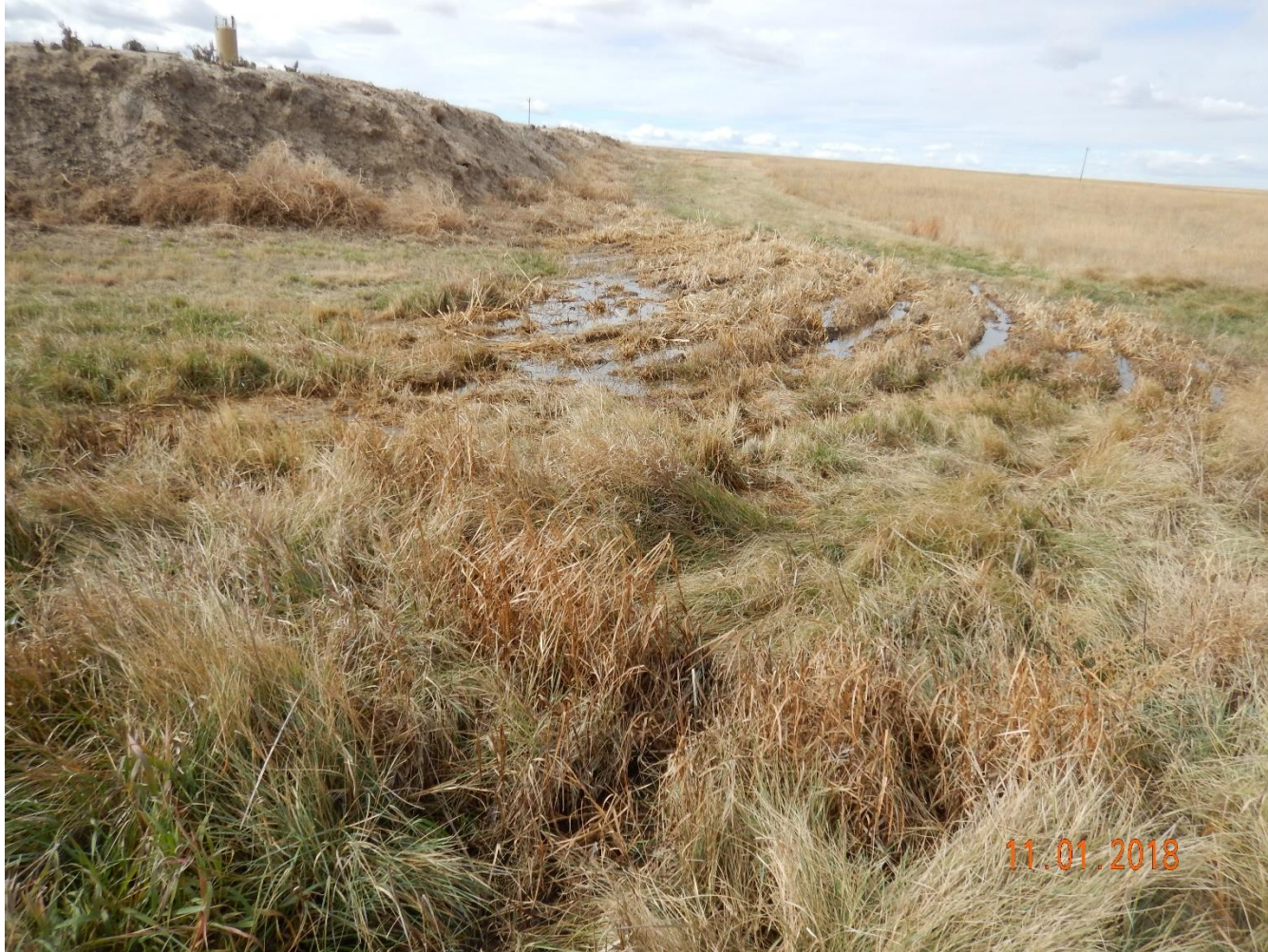
Photo 20: Photo taken from the east of the pit facing west. Photo shows produced water being discharging from the base of the pit.
