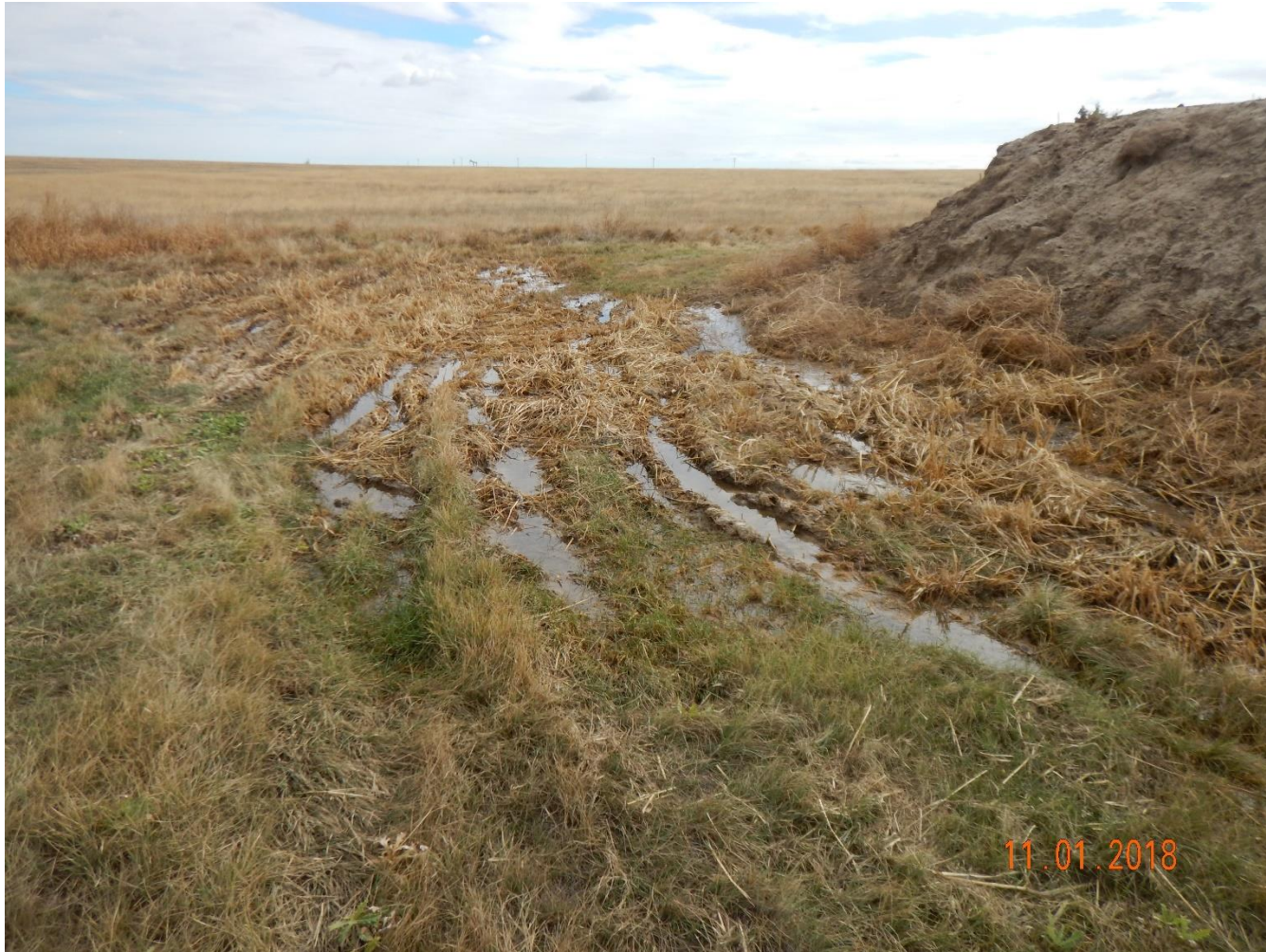
Photo 18: Photo taken from the northeast end of the pit facing east. Photo shows produced water being discharging from the base of the pit.
