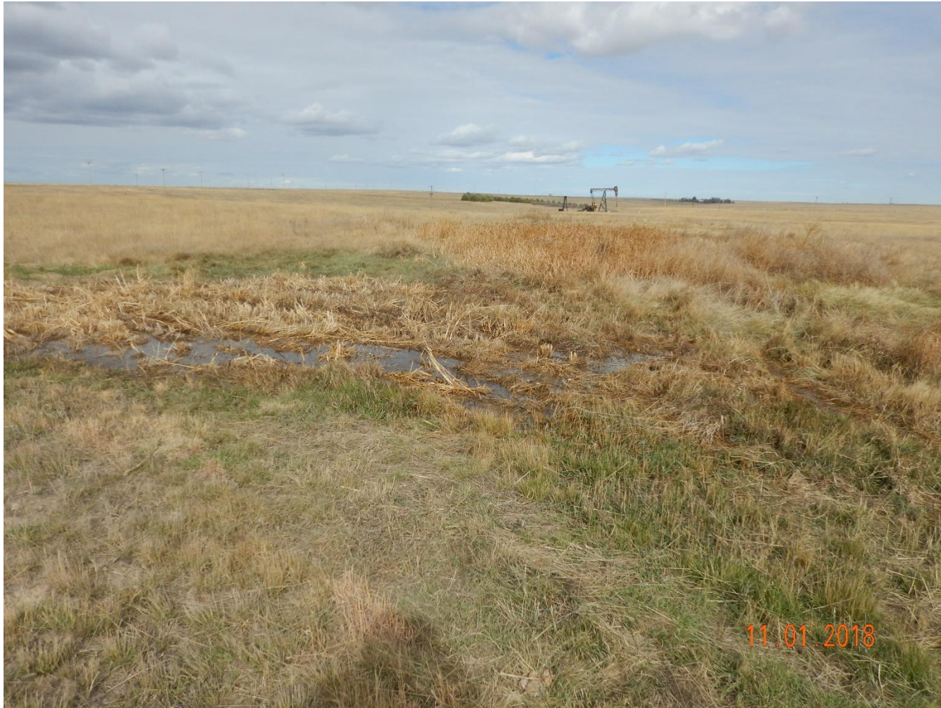
Photo 21: Photo taken from the east of the pit facing north. Photo shows produced water being discharging from the base of the pit.
