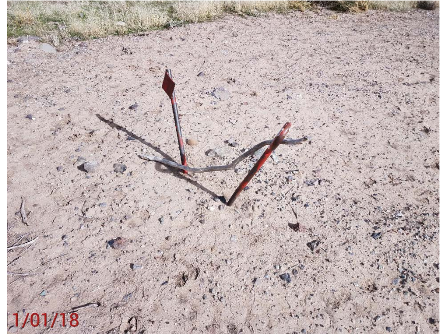
Location Photo #6, improperly marked deadman
