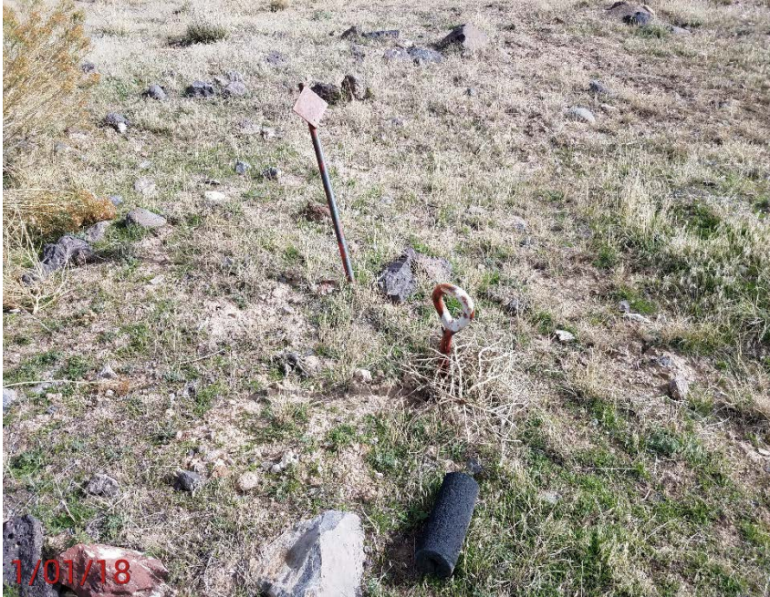
Location Photo #7, improperly marked deadman
