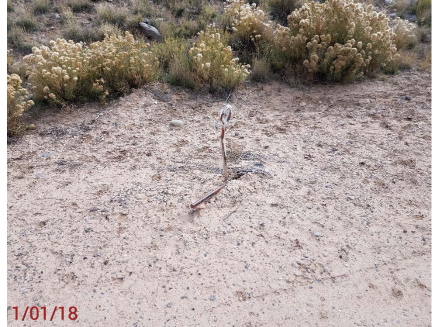
Location Photo #8 , improperly marked deadman
