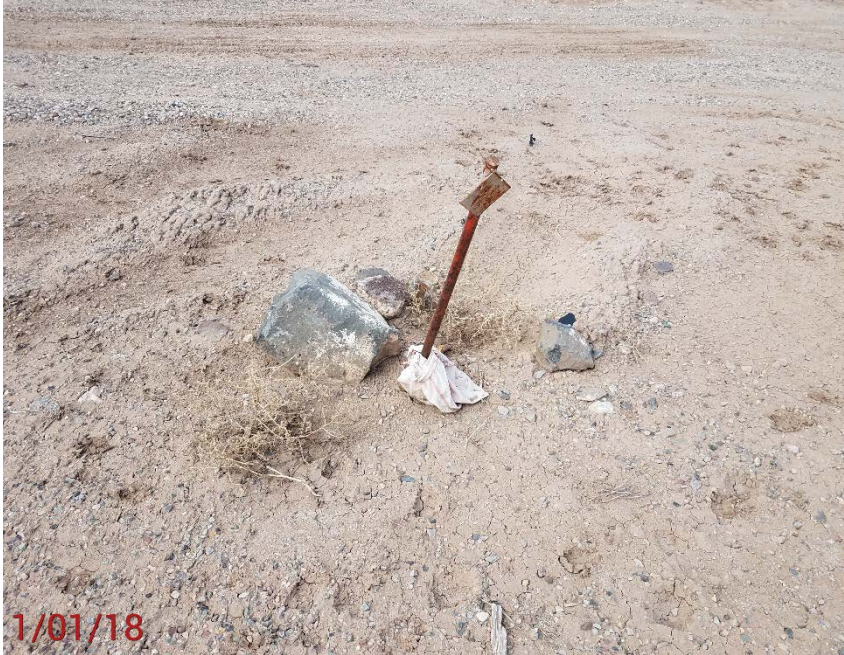
Location Photo #9 , improperly marked deadman
