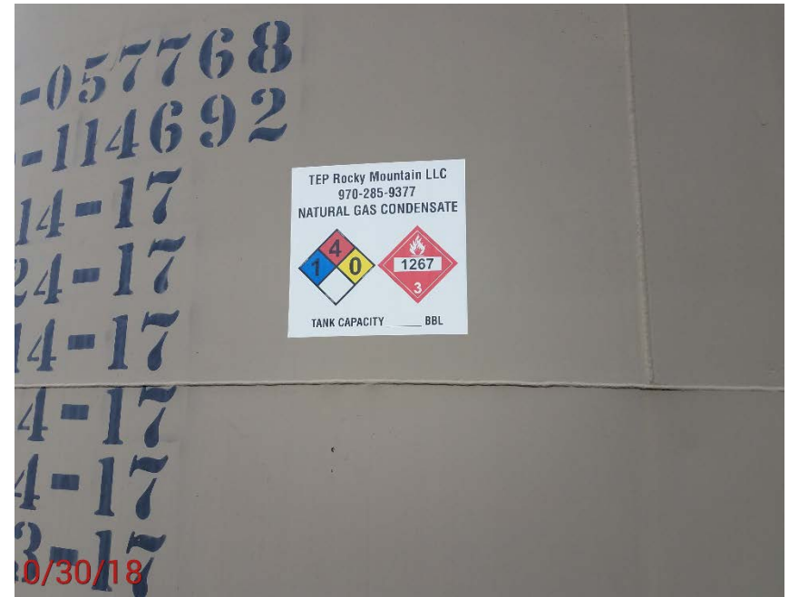
Location Photo #6, Missing capacity on all tanks
