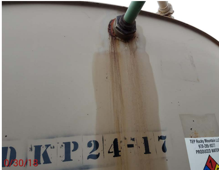
Location Photo #5, Mechanical condition of tank fitting.
