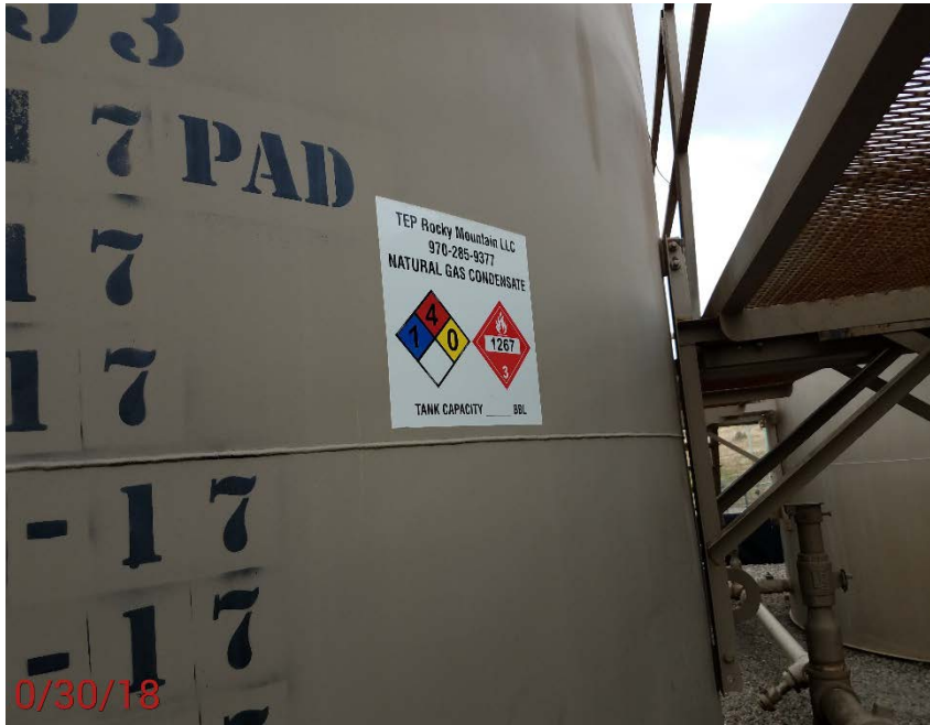
Location Photo #7, Missing capacity on all tanks
