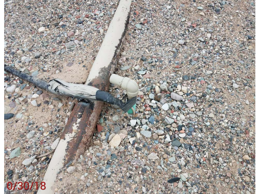
Location Photo #4, Unmarked flow line.
