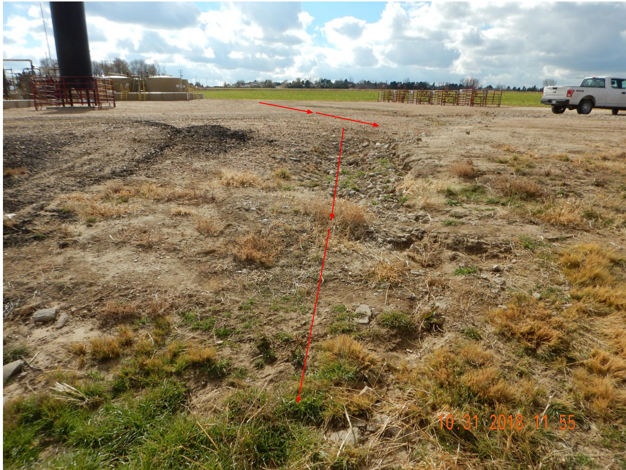
Photo 6. Photo taken from the northern location, facing South. Photo illustrates stormwater runoff from location with the evidence of an erosion channel.
