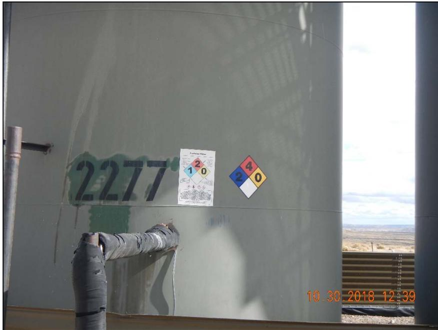
Photo 3. Faded tank capacity.
