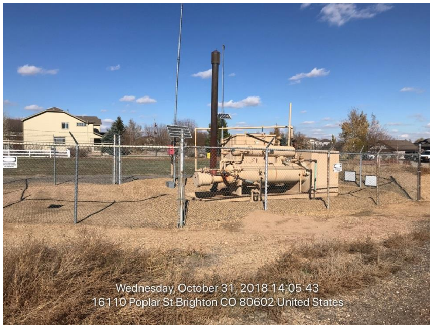
Photo#3 Separator and Gas Meter
