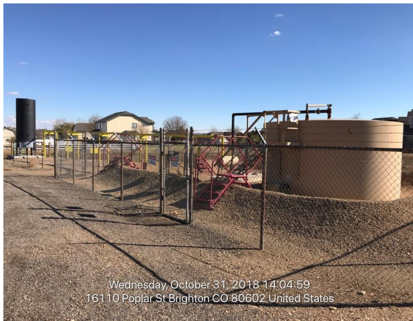
Photo#1 Production tank/Produced water pit/ECD
