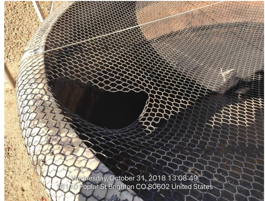
Photo#4 Corrective Action/Repair netting over produced water pit
