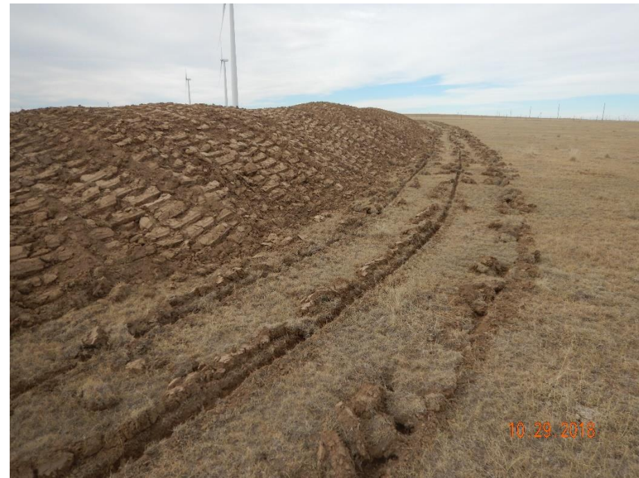
Photo 6: Photo taken from the northeast corner of the location, facing west. Photo shows surface roughening has been used as a perimeter stormwater and erosion control BMP. Photo also shows topsoil pile on the south end of the location.
