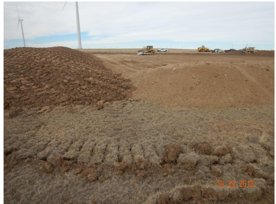
Photo 4: Photo taken from the southeast end of the location, facing west. Photo shows operator has segregated the topsoil pile (left) and a "B" horizon (right).
