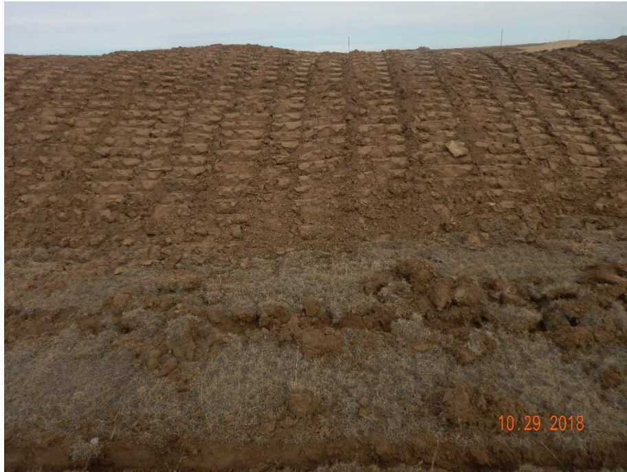
Photo 3: Photo taken from the south end of the location, facing north. Photo shows topsoil pile has been tracked.
