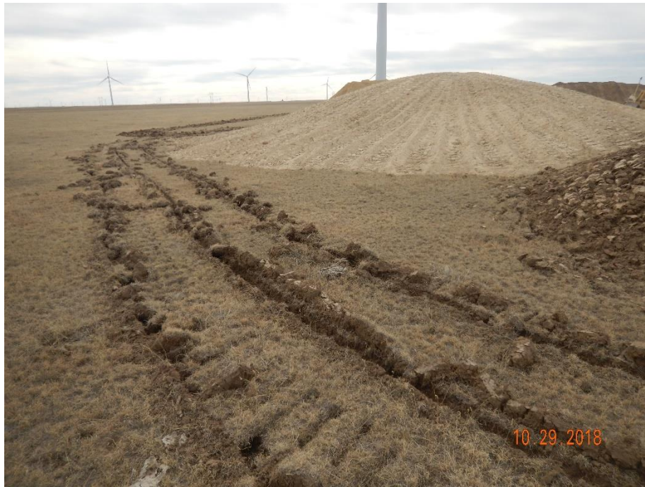
Photo 5: Photo taken from the northeast corner of the location, facing south. Photo shows surface roughening has been used as a perimeter stormwater and erosion control BMP. Photo also shows subsoil stockpile on the east end of the location.
