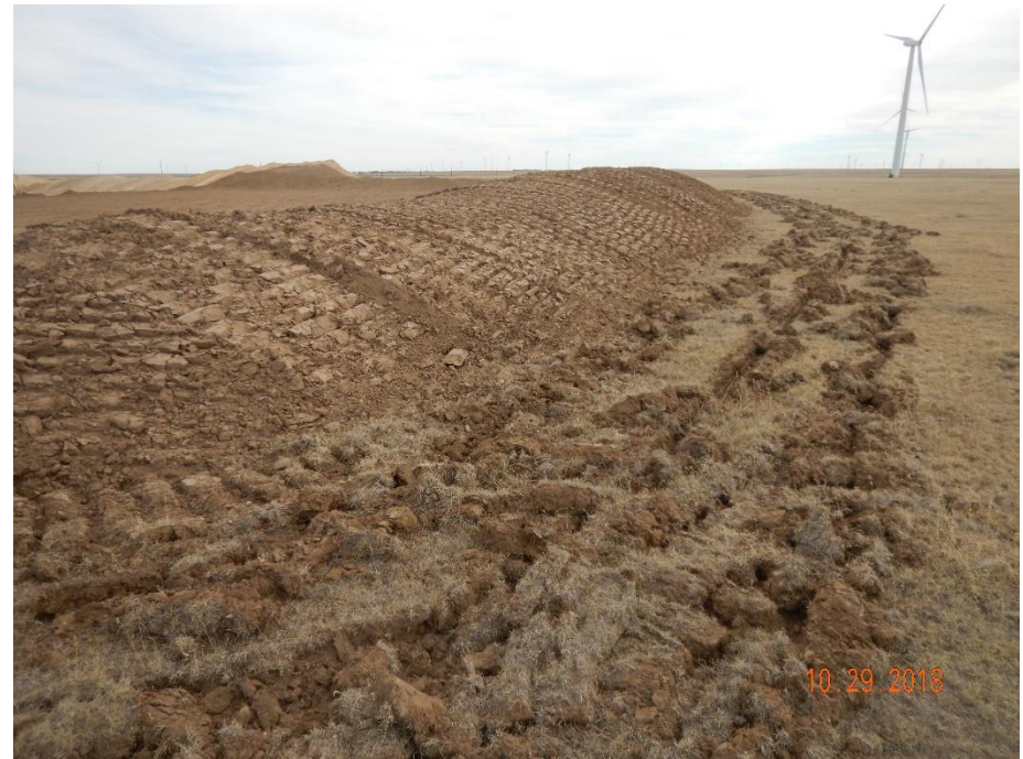
Photo 2: Photo taken from the southwest corner of the location, facing east. Photo shows surface roughening has been used as a perimeter stormwater and erosion control BMP. Photo also shows topsoil pile on the south end of the location.
