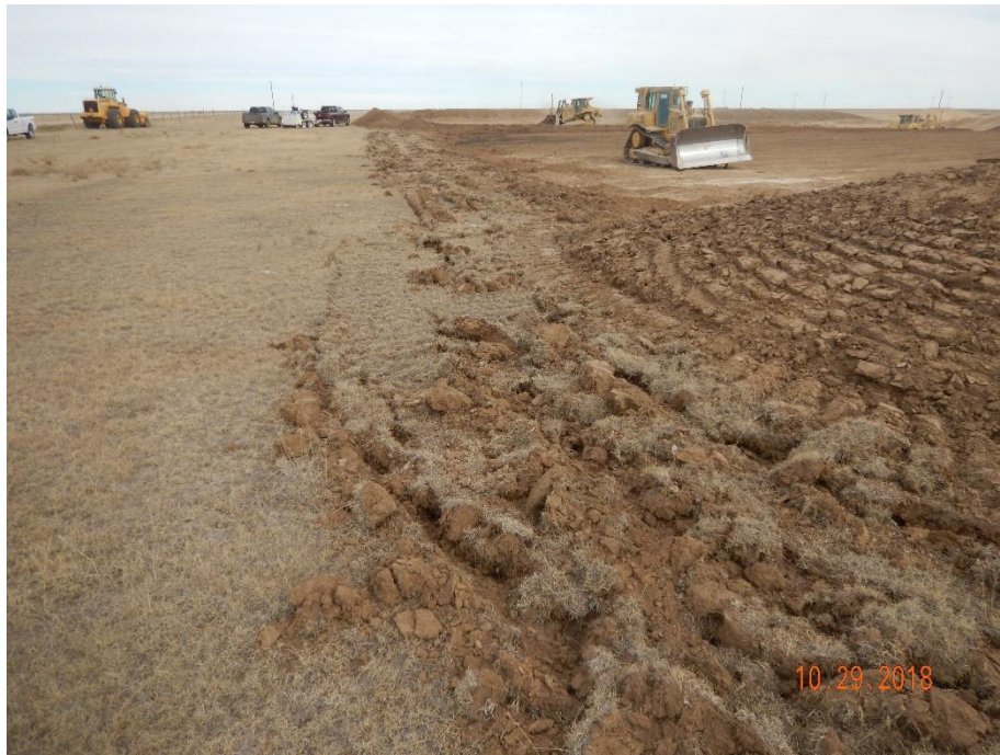
Photo 1: Photo taken from the southwest corner of the location, facing north. Photo shows surface roughening has been used as a perimeter stormwater and erosion control BMP. Photo also shows topsoil pile on the south end of the location.
