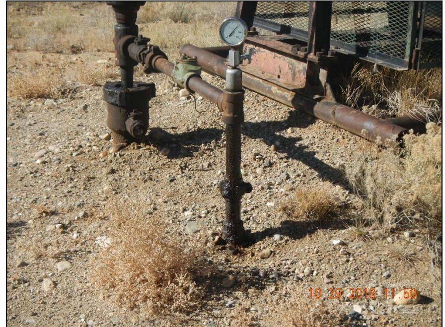
**Photo 2. Stained soil/leak at wellhead.**
