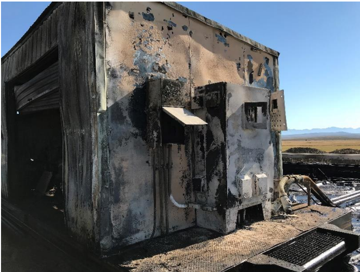
Photo of C7 Pump House south wall with Power Panel Box in center, low voltage breaker box to left and PLC box to right. Power lines enter the Power Panel Box from the cable tray to the far right.
