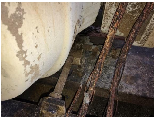
Enlarged view of ground wire to motor base connection and adjacent power lines.
