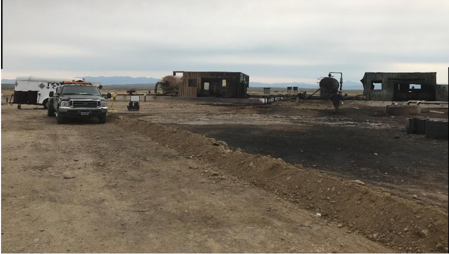
Photo 1: Wellpad View looking east at C8 and C7 Pump Houses, left to right Soot fallout inside and outside of containment dike is visible
