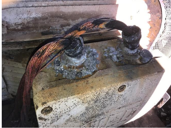
Power In to C7 Triplex 200hp Motor Connection
