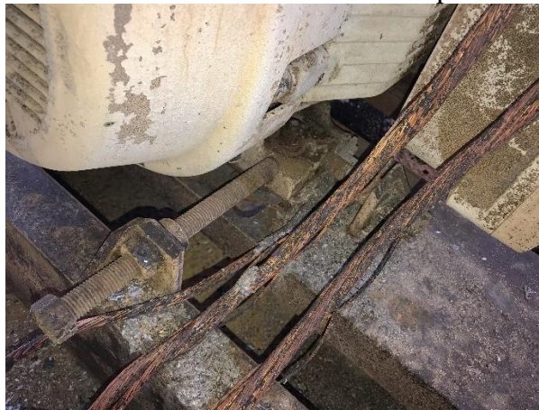
C7 Skid Pass Through Power Lines and Ground Line 200hp Motor
