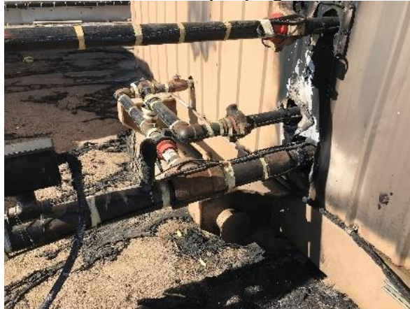
C5 Close up photo of pump piping and wall soot marks
