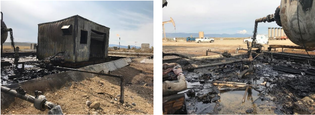
Damaged C7 Pump House, Separator with damaged suction hose and hydrocarbons inside containment
