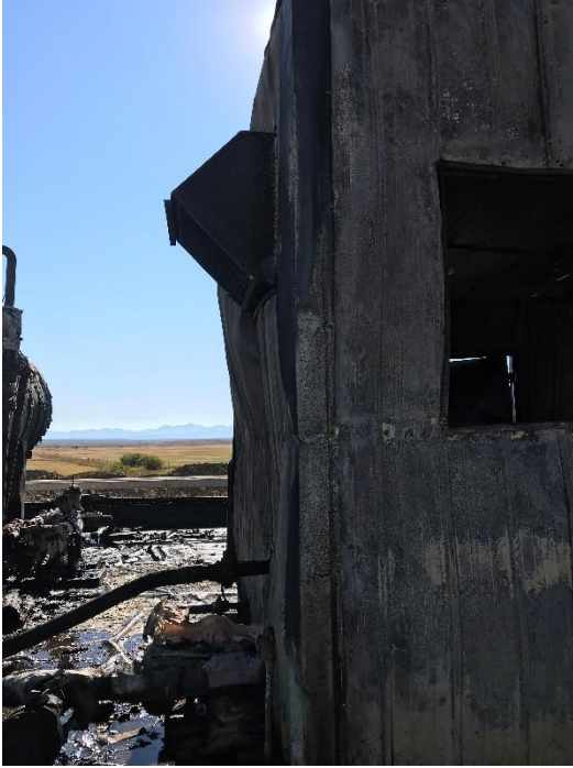
Photo of C7 Pump House north wall deformation facing the horizontal separator. The discharge line is above the suction line connect at this wall in the foreground.
