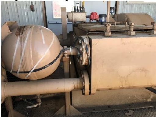
C5 Discharge Line above Suction Line out/in of C5 Pump Triplex Pump Top Inspection Cover and handle is visible in background
