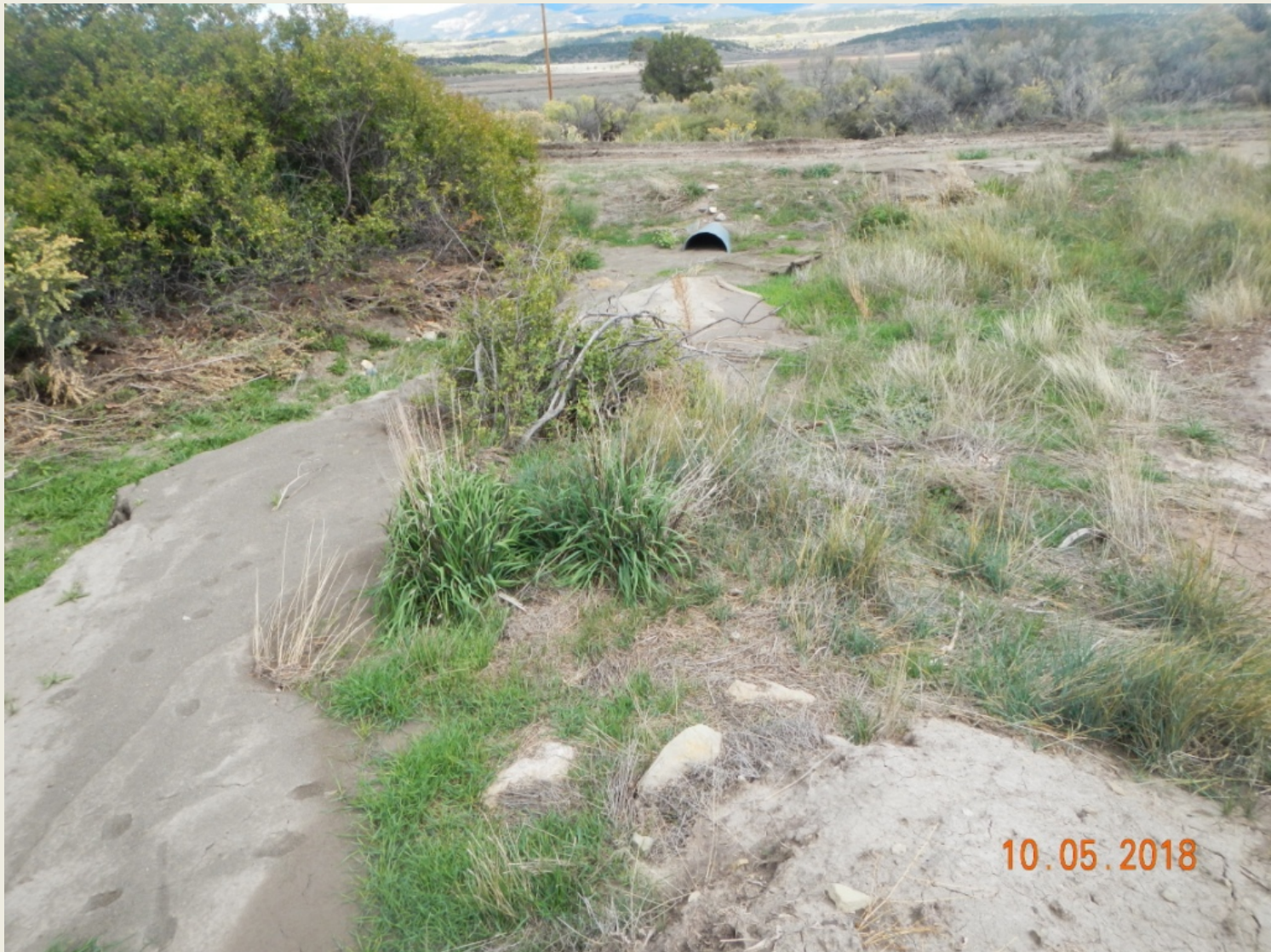
Photo 5. View of area in the northwestern project area where diverted stormwater flows toward a culvert leading off of the project area. Sediment is not being properly managed. Culvert is half full of sediment.
