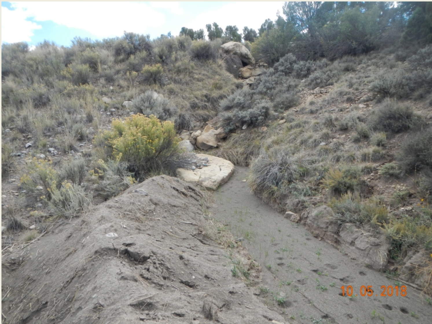
Photo 3. View of the area in the southwestern corner of the project area where it appears that stormwater and sediment flows onto the project area toward the western diversion.
