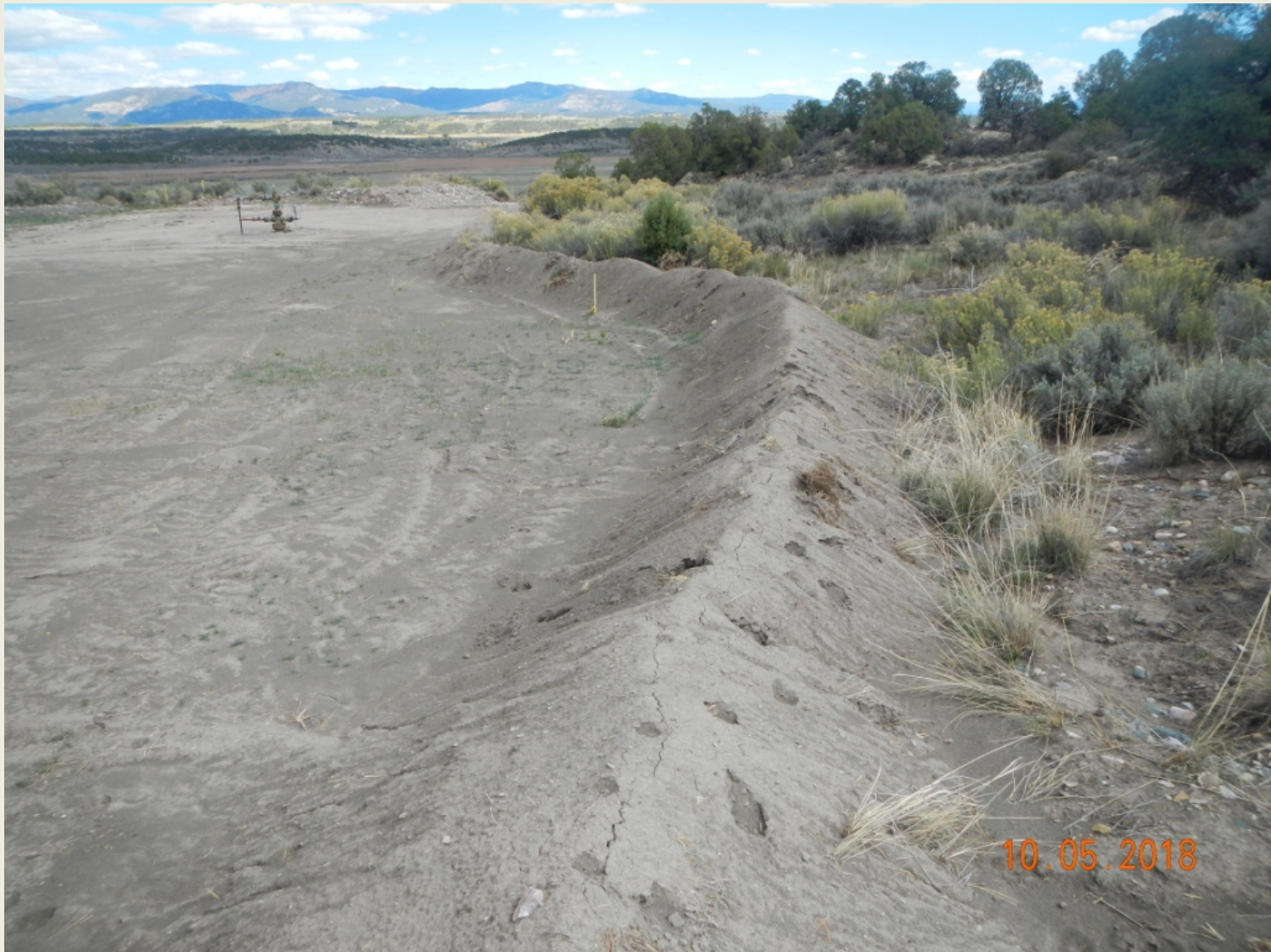
Photo 6. View of the southern project area from the southwestern corner facing eastward. Berms are not properly stabilized.
