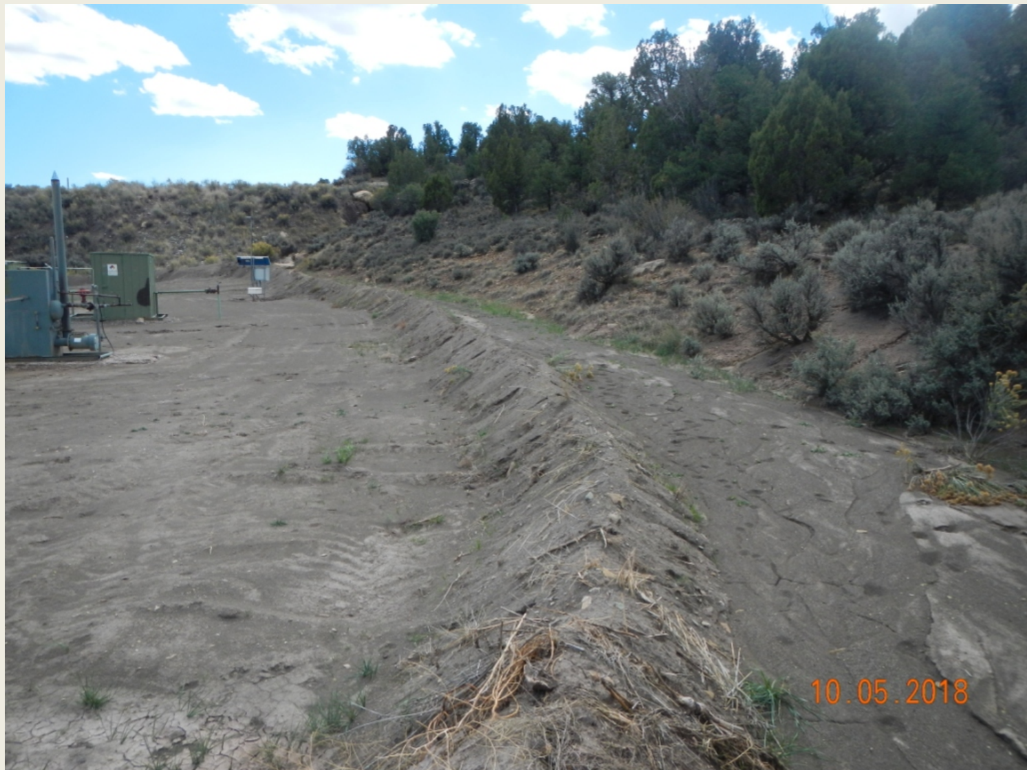
Photo 2. View of the western project area from the northwestern corner facing southward. Berms are not stabilized and diversion is full of sediment.
