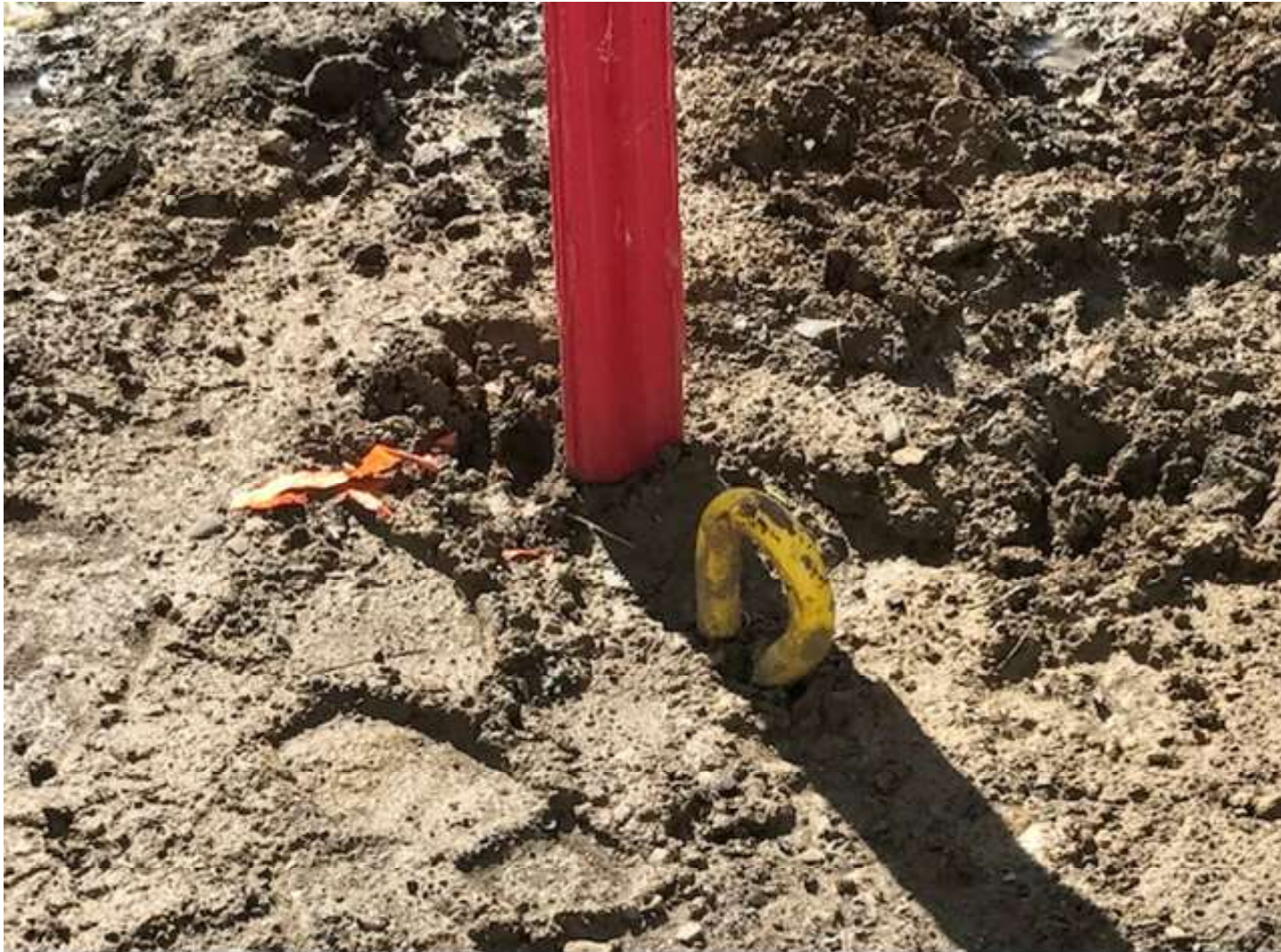
A NEW MARKER WAS INSTALLED ON THE UNMARKED DEADMAN ANCHOR IN COMPLIANCE WITH RULE 604.c.Q.
