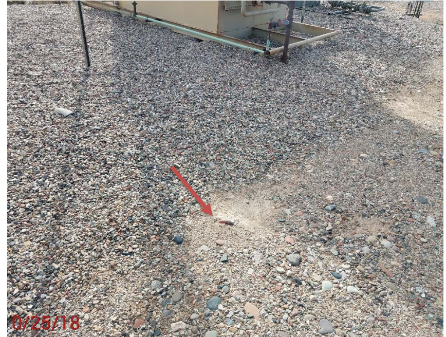
Location Photo #4, unmarked deadman near separator
