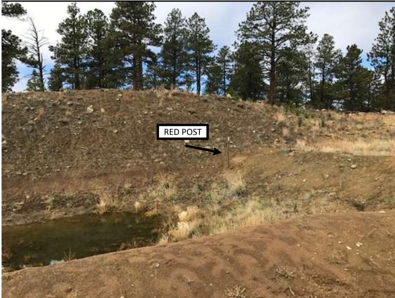
A POST WAS INSTALLED IN THE PRODUCTION PIT TO MONITOR (2) FOOT OF FREEBOARD BETWEEN THE TOP OF THE PIT WALL AND THE FLUID LEVEL OF THE PIT.
