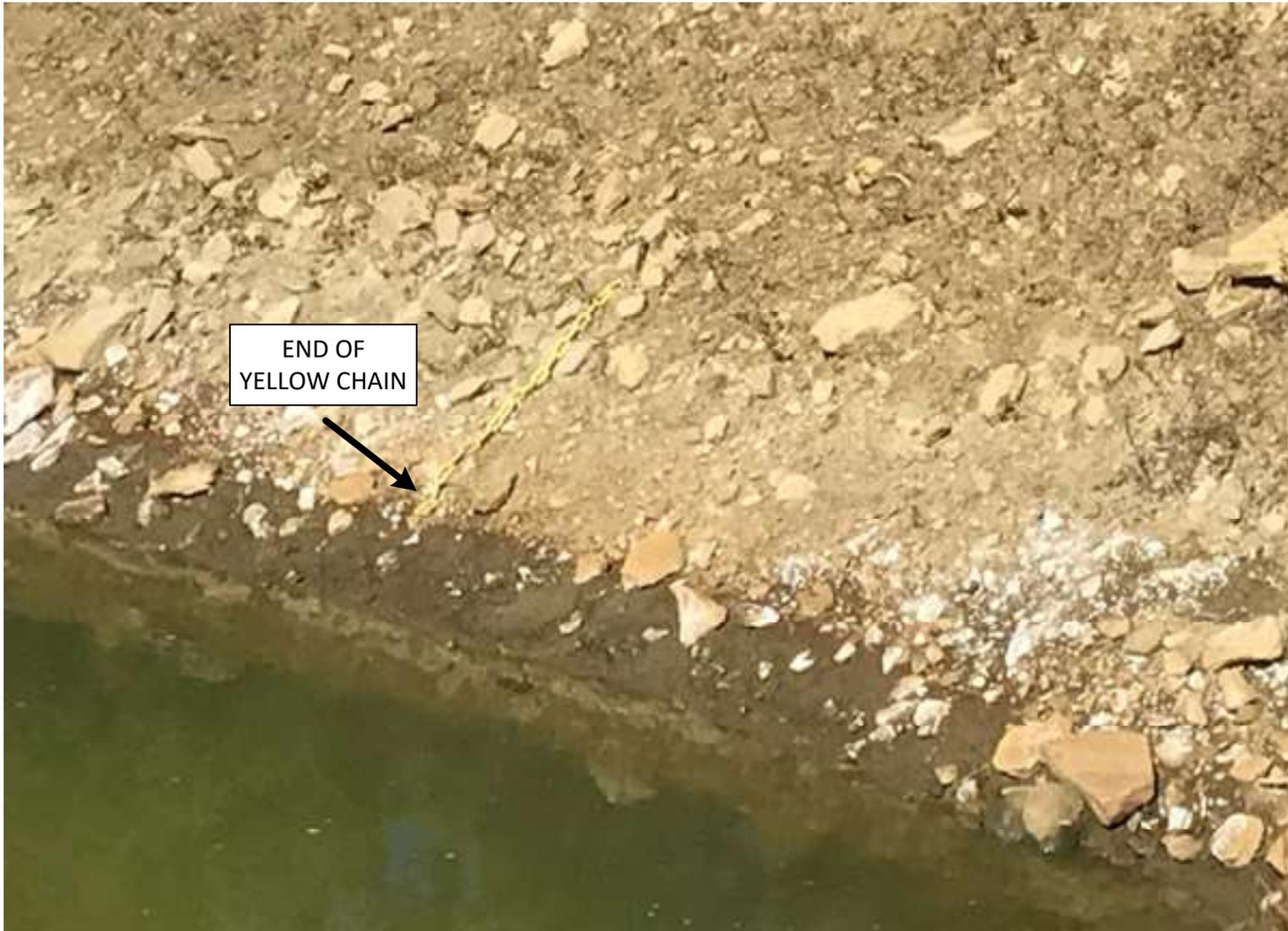
THE PRODUCED WATER WAS PULLED FROM THE PRODUCTION PIT TO PROVIDE (2) FEET OF FREEBOARD, IN COMPLIANCE WITH RULE 902.B.
